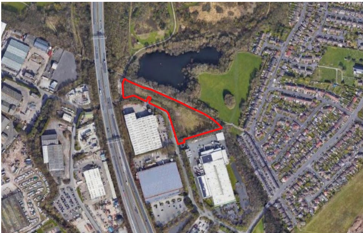
Figure 2 Satellite image showing the red site boundary of the whole site.
