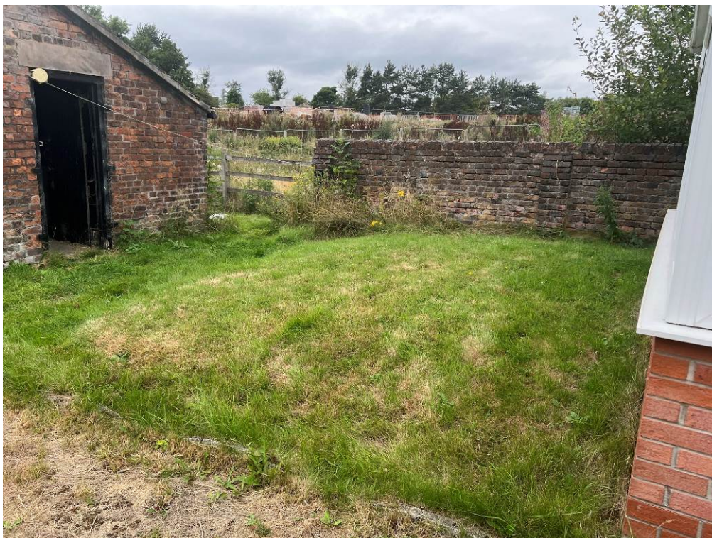
Photo 4; Outbuilding and wall to the side of Dye House.
