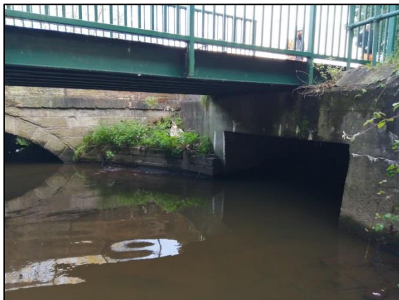
View under road and pedestrian bridge at confluence of Simonswood Brook and unnamed tributary – no suitable ledges for riparian mammal use.
