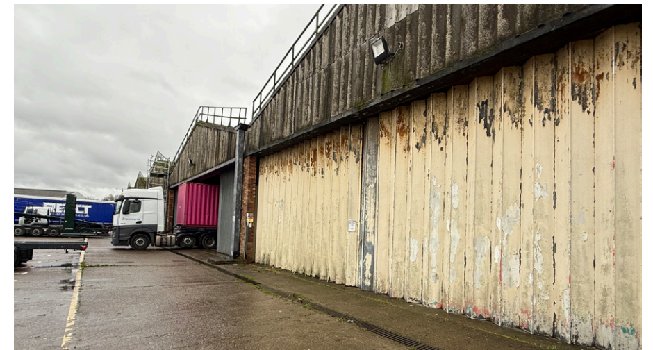
Tired/dated existing warehouse building on site
