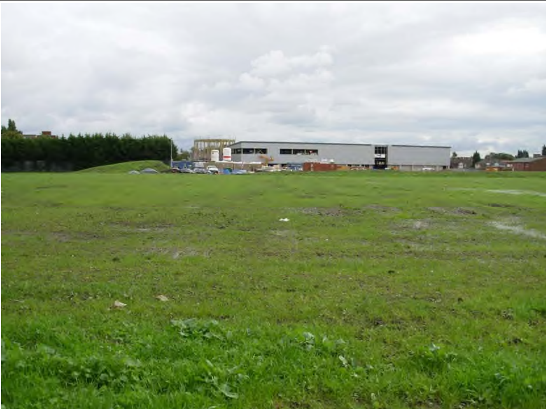
Photo 18: View east through railings showing construction site
