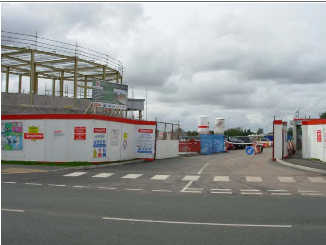
Photo 20: View west of site entrance to construction site
