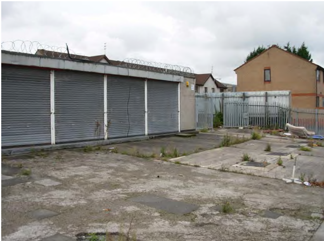
Photo 25: View southwest of derelict garage building off Cherryfield Drive
