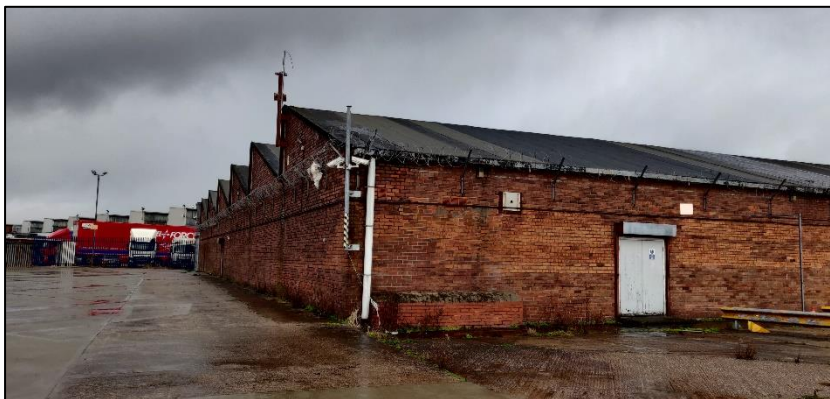
Photograph 24 showing the roof of the smaller warehouse
