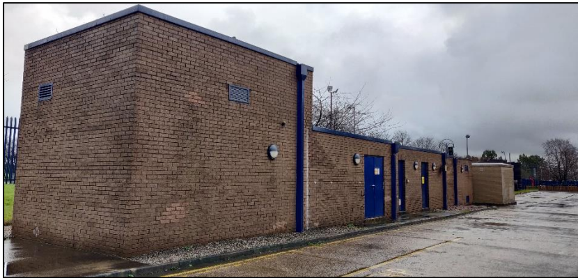
Photograph 30 showing the single-storey building
