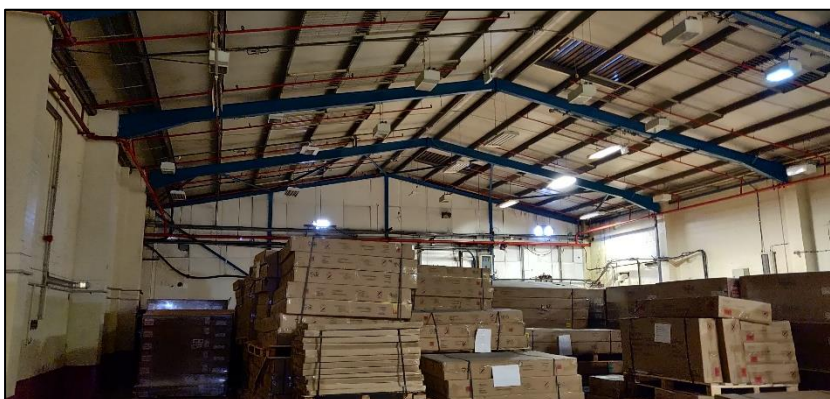
Photograph 18 showing another of the large internal spaces
