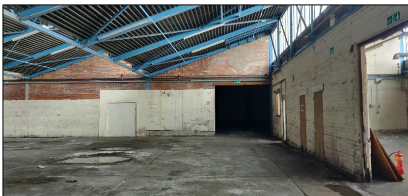
Photograph 26 showing another section of the smaller warehouse internally
