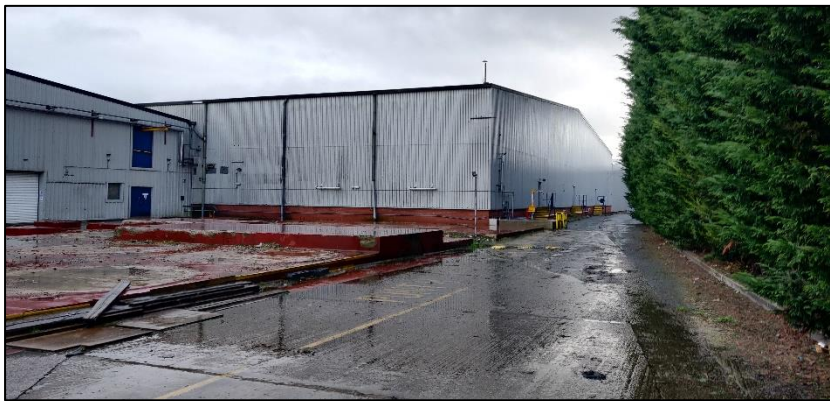
Photograph 14 showing the corrugated metal panels covering the entire rear walls
