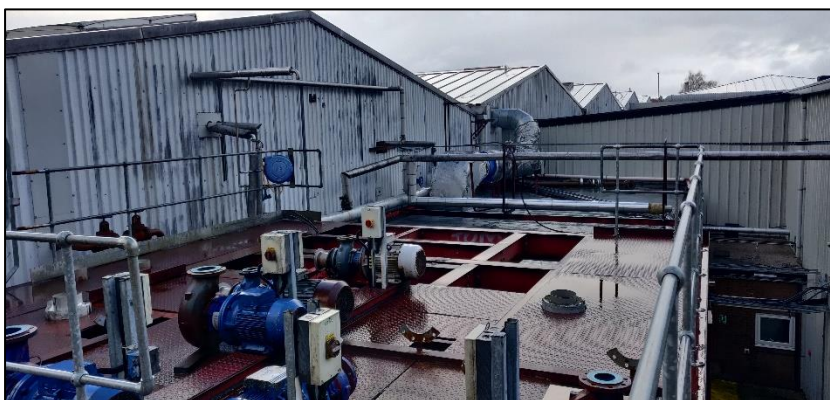
Photograph 15 showing some sections of the roof at the rear of the building
