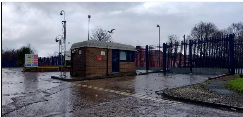
Photograph 31 showing the gate hut
