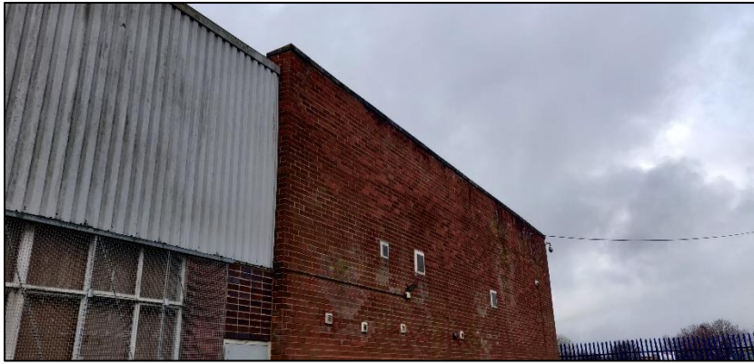
Photograph 22 showing the section of metal cladding
