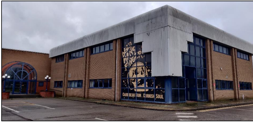
Photograph 13 showing the corrugated metal panel on the upper walls
