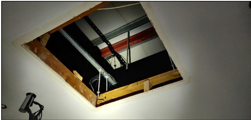
Photograph 20 showing the space above one of the offices
