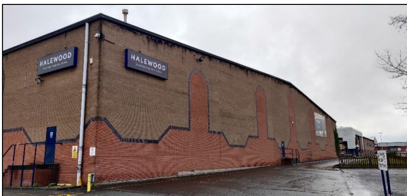
Photograph 12 showing the exterior brickwork
