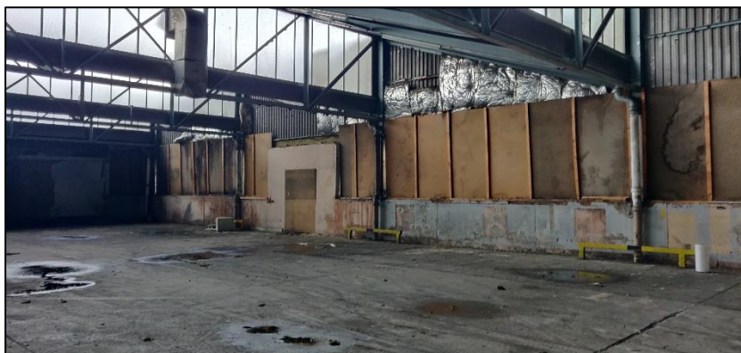
Photograph 25 showing the interior space of the smaller warehouse
