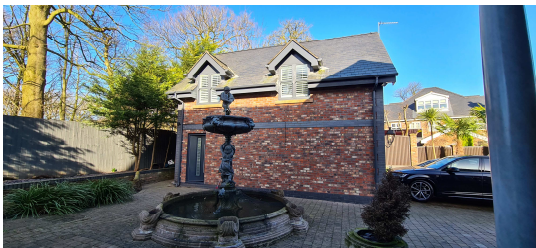
Figure 07 External photograph of the detached outbuilding to 4 High Carrs. Taken Feb 2021.
