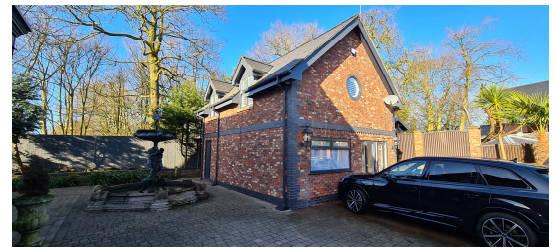
Figure 08 External photograph of the detached outbuilding to 4 High Carrs. Taken Feb 2021.
