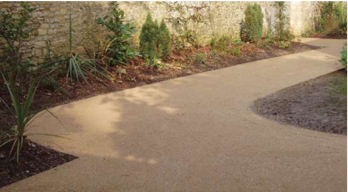
Pathways - Self Binding Gravel (In keeping with the rest of the site)
