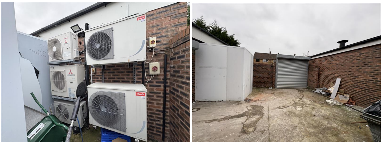
Figure 1: Photograph of current Ground Floor plant area, behind timber boarding.
