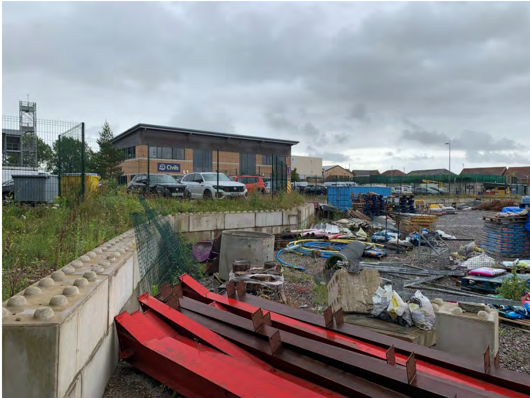
Strip of bare ground along the edge of the site.
