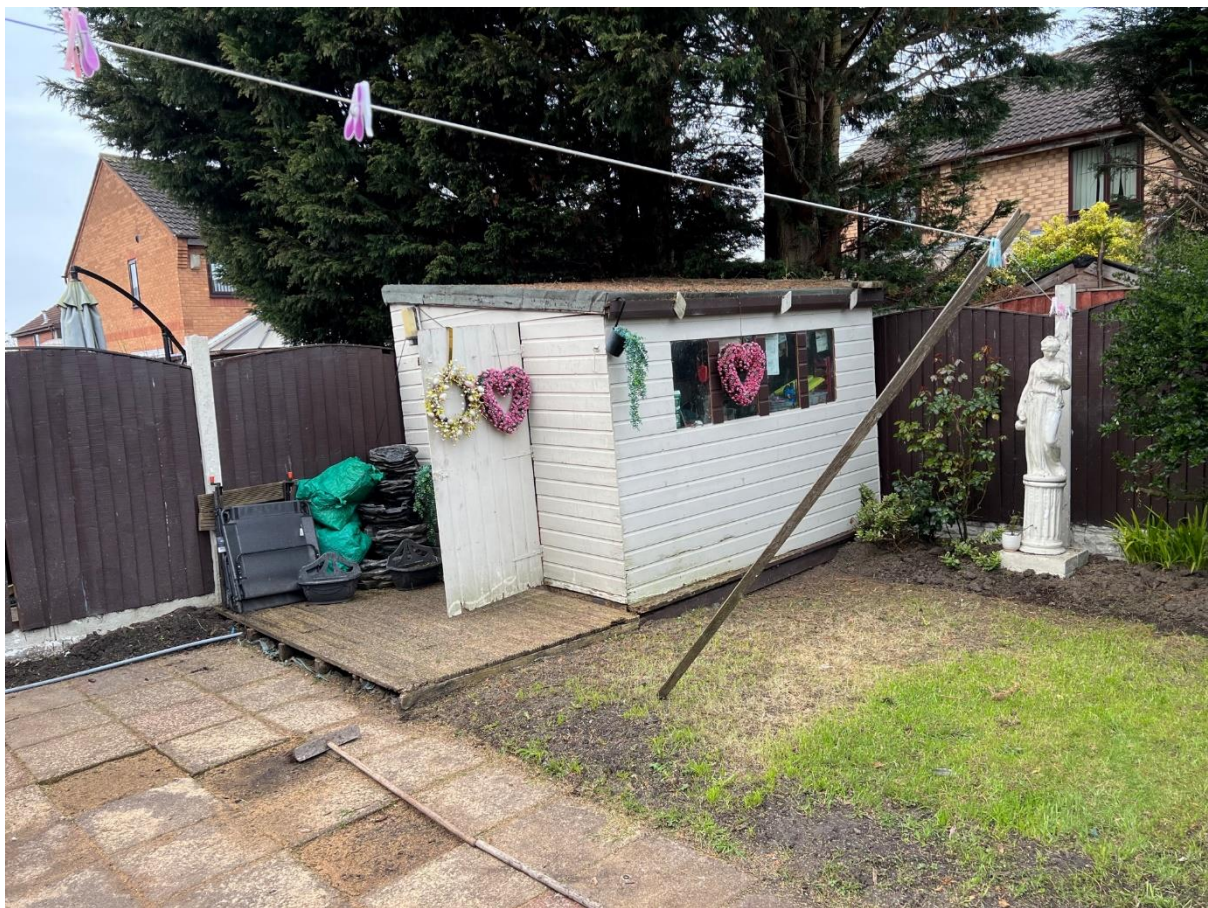
Garden shed and apron with plastic vapour barrier beneath. Hard paving to front of existing conservatory.
