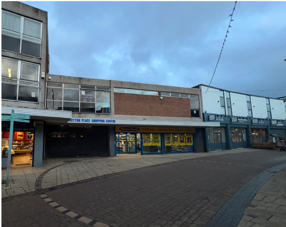
02. Existing neighbouring retail unit
