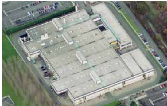
06. Interchange Motorway Industrial Estate
