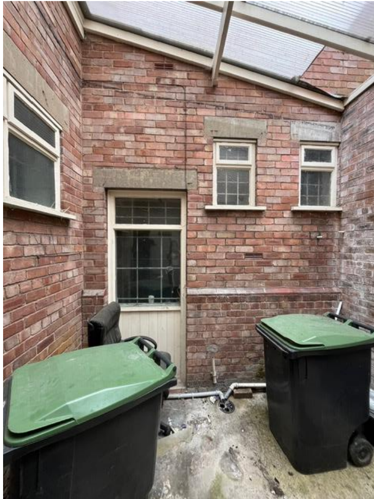
Yard area where the extract will be installed
