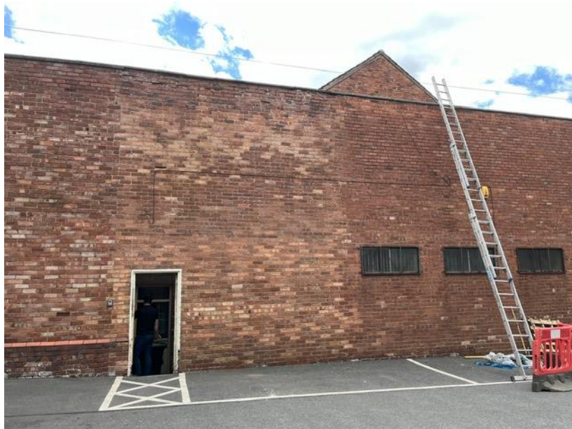
Wall to the rear of the building
