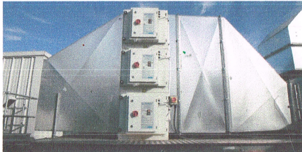
3 ESP Units Stacked in modular formation
