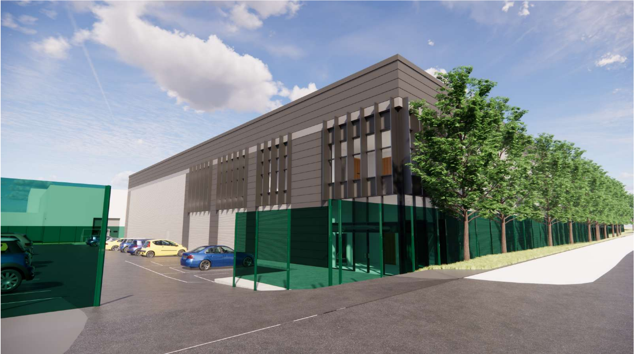
STREET VIEW LOOKING FROM CAR PARK ENTRANCE TOWARDS OFFICE
