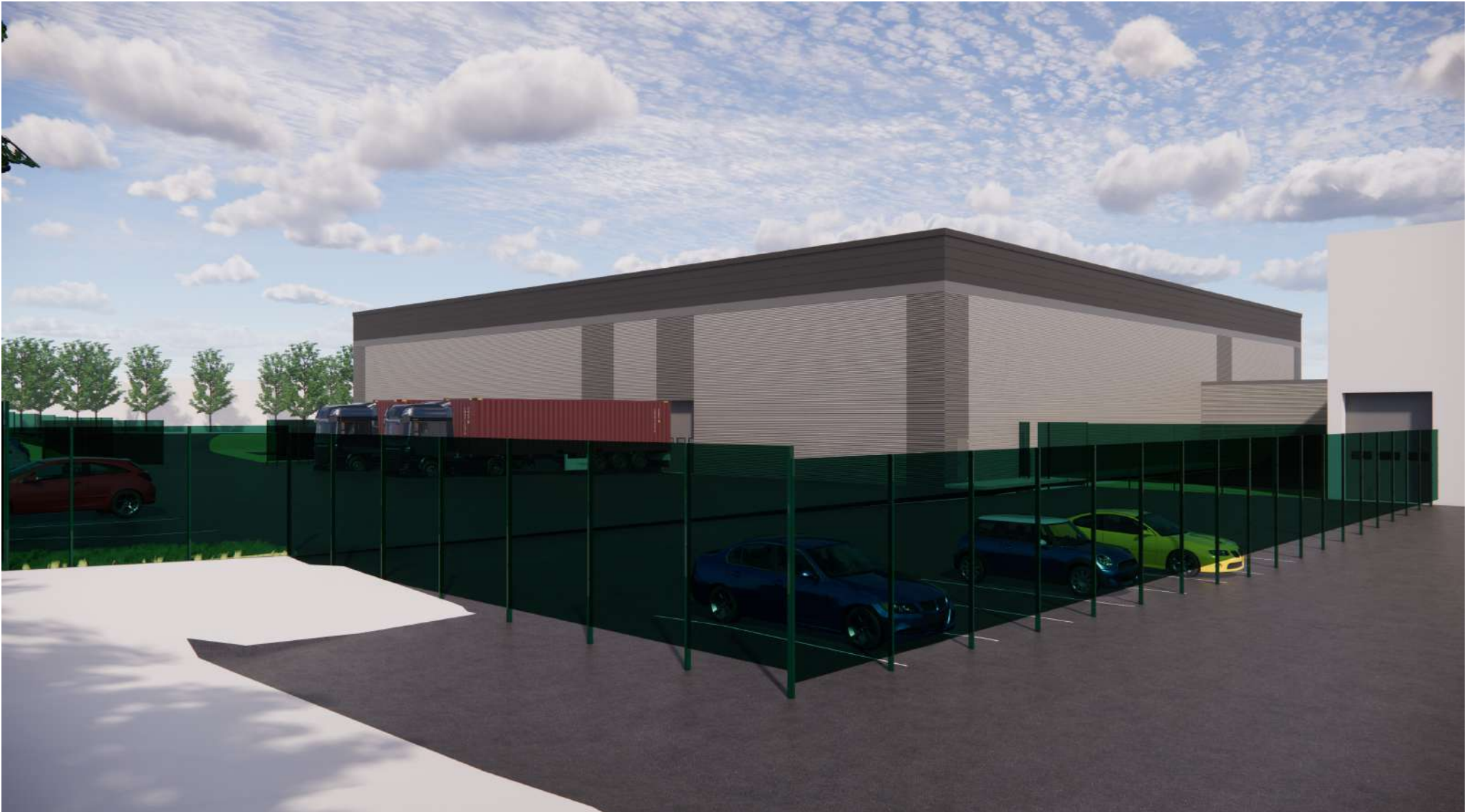
STREET VIEW LOOKING FROM NEXUS HOUSE SERVICE YARD TO BUILDING
