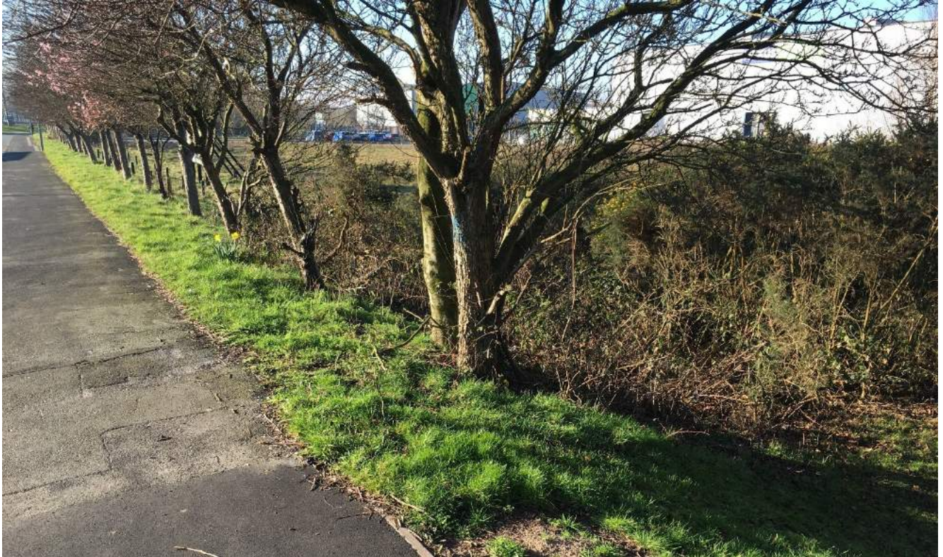
Banking along boundary with Gellings Road.
