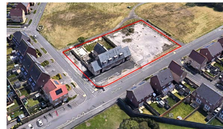
Aerial Photo overlooking the existing public house
