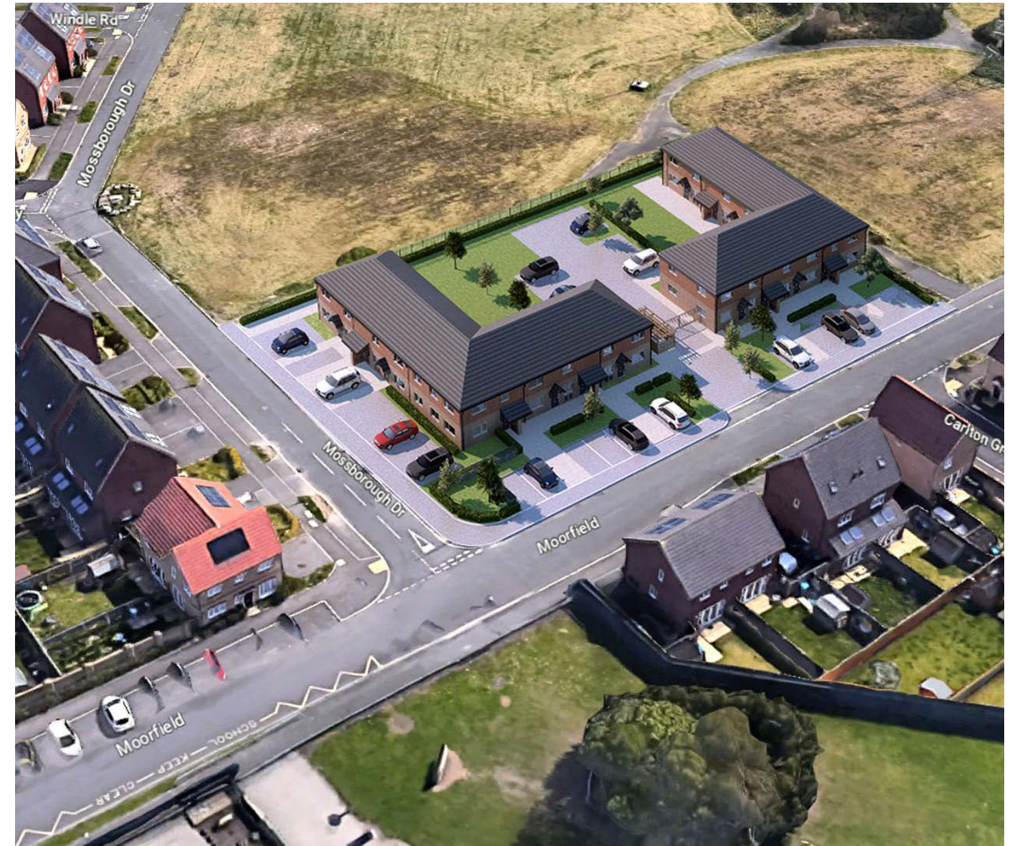
Aerial view over the development
