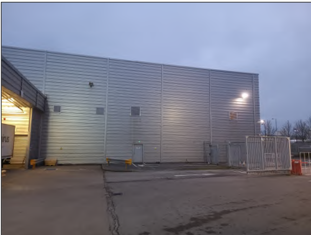
Photo Plate No. 05: View of western side of building (Looking Southeast).
