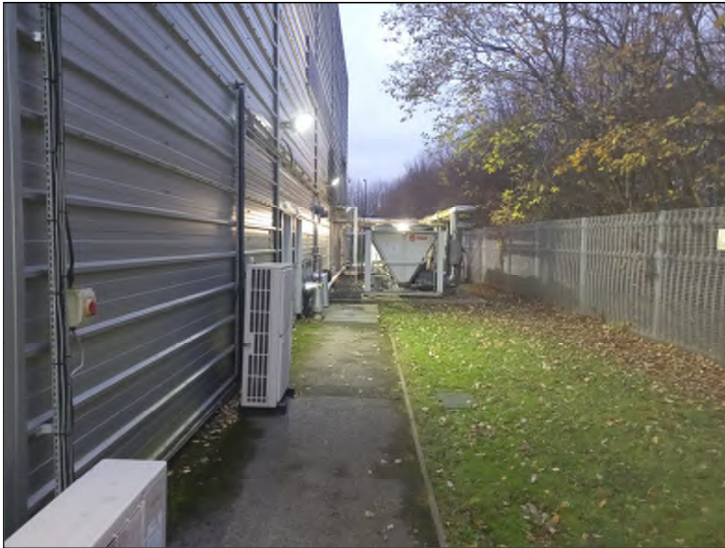
Photo Plate No. 01: View of northern site boundary and plant connecting to northern side of building (Looking West).
