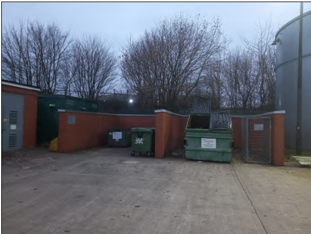
Photo Plate No. 07: Refuse area in the Western part of the site.
