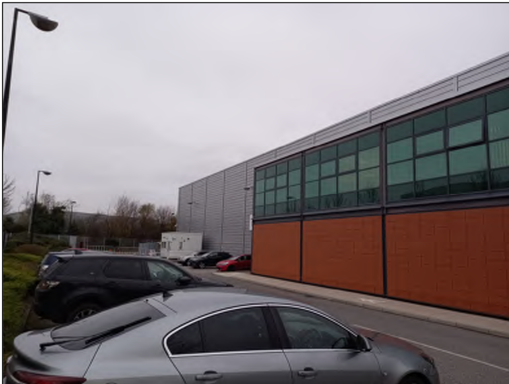
Photo Plate No. 03: View of southern side of building (Looking Northwest).
