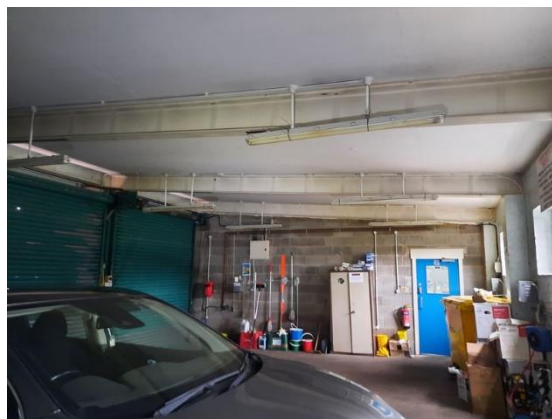
Plate 4.5: South-east Section of Building B1.
