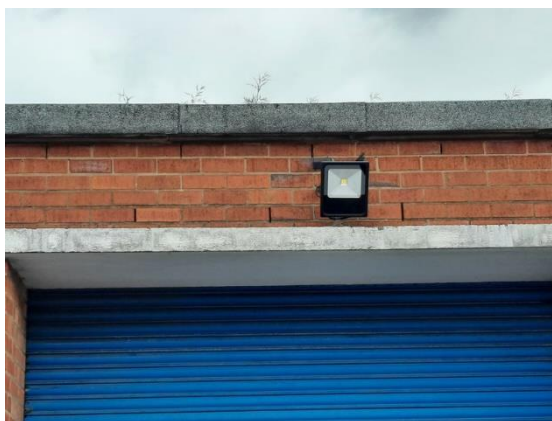
Plate 4.3: Weep Holes and Security Light Above Concrete Porch at South End of South-west Elevation of Building B1.
