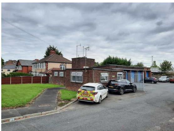
Plate 4.1: Building B1 from North-west Viewpoint.
