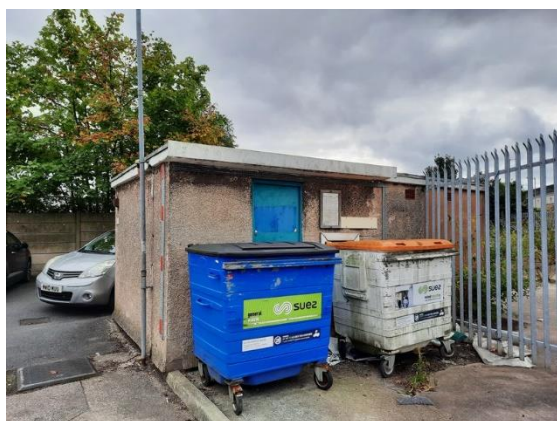
Plate 4.6: North-west Elevation of Building B2.
