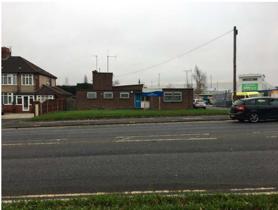
Plate 2: Looking south-east across Archway Road at the existing Ambulance Station located within the north-eastern part of the Site.
