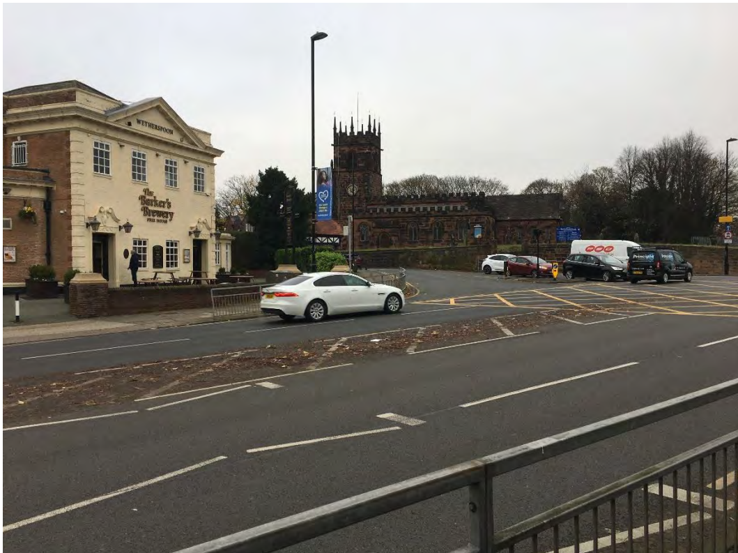
Plate 10: Looking from the former junction of Derby Road with Archway Road and Blue Bell Lane north towards the Church of St Michael.
