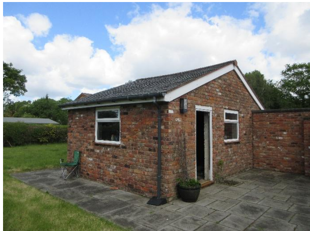
Photo 22: Western and southern elevations of the garage
