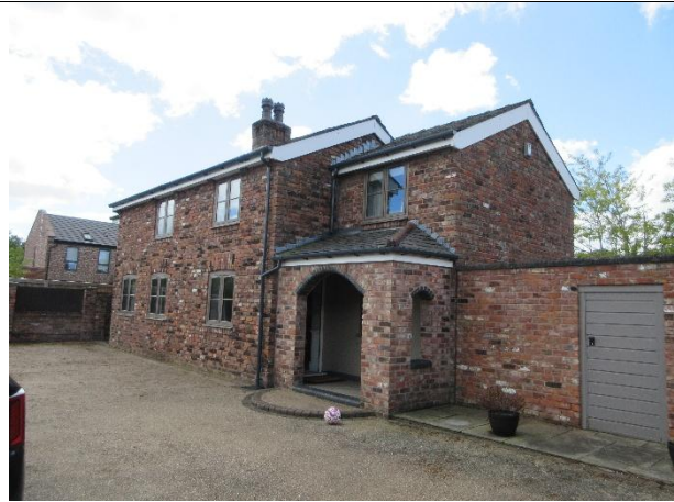
Photo 14: Eastern and northern elevations of the house
