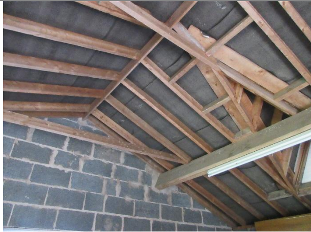
Photo 26: Interior of garage
