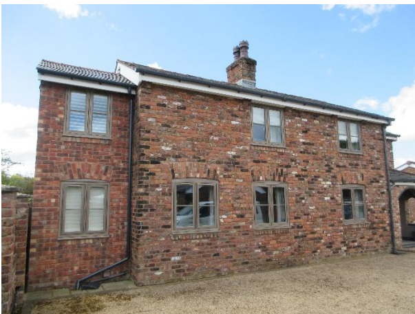
Photo 15: Eastern elevation of the house
