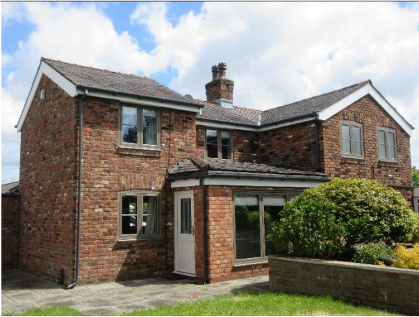
Photo 13: Northern and western elevation of house
