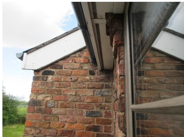
Photo 16: Sealed PVC fascia and soffits at the house
