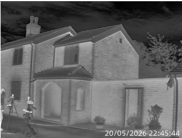
Photo 31: NVA view at Survey Position 1 (House)
