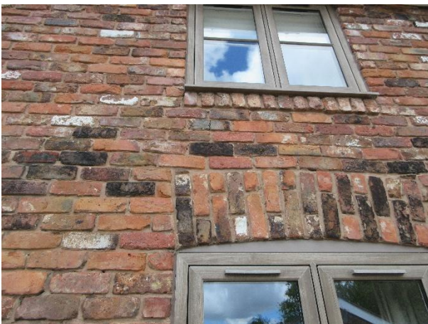
Photo 17: Pointed brickwork at the house and no gaps at window frames
