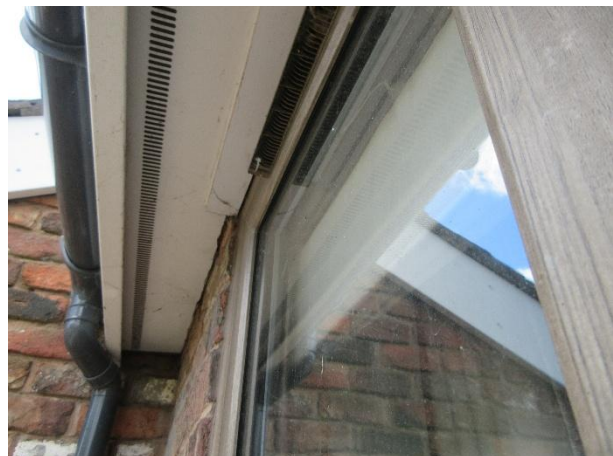
Photo 18: Sealed soffits at the house
