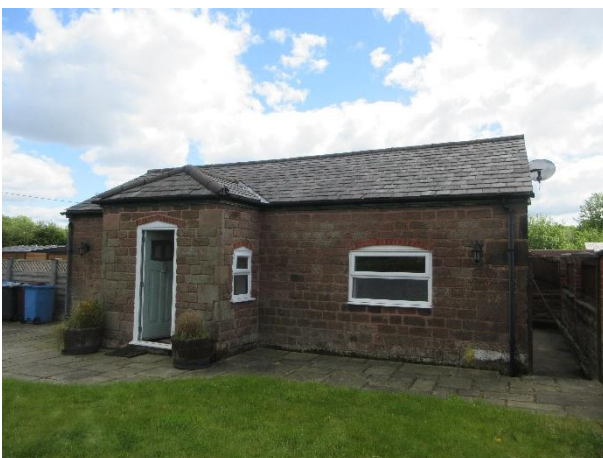
Photo 5: Northern elevation of cottage
