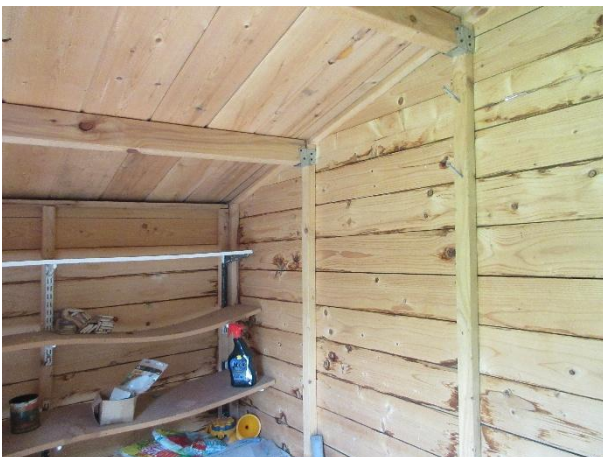
Photo 29: Interior of Shed 1
