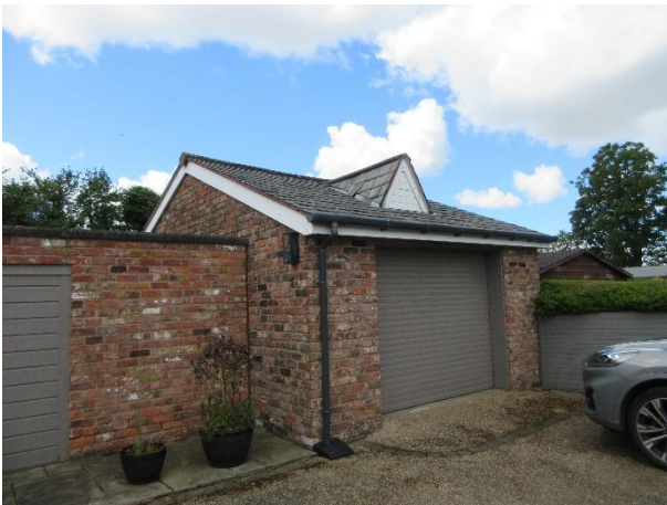
Photo 21: Wall and southern and eastern elevations of the garage
