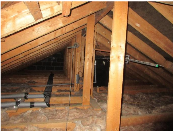
Photo 11: Roof void at cottage
