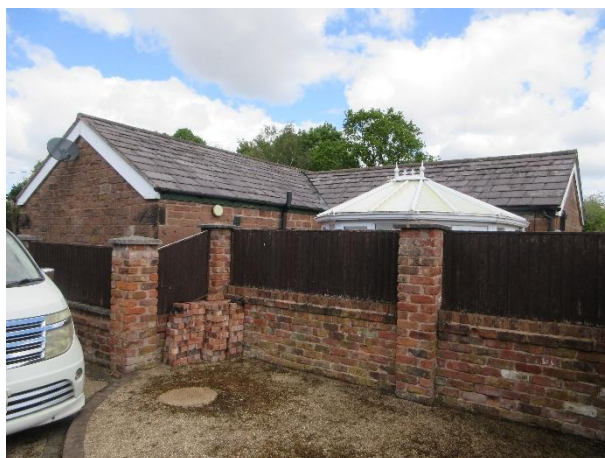
Photo 6: Western and southern elevations of cottage
