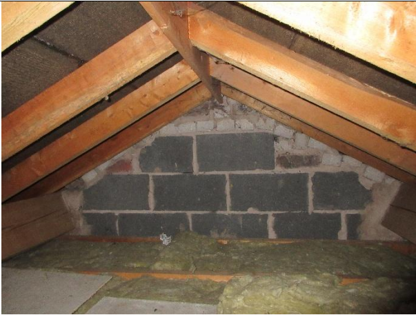
Photo 19: Roof void at the house
