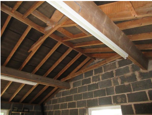
Photo 27: Interior of garage
