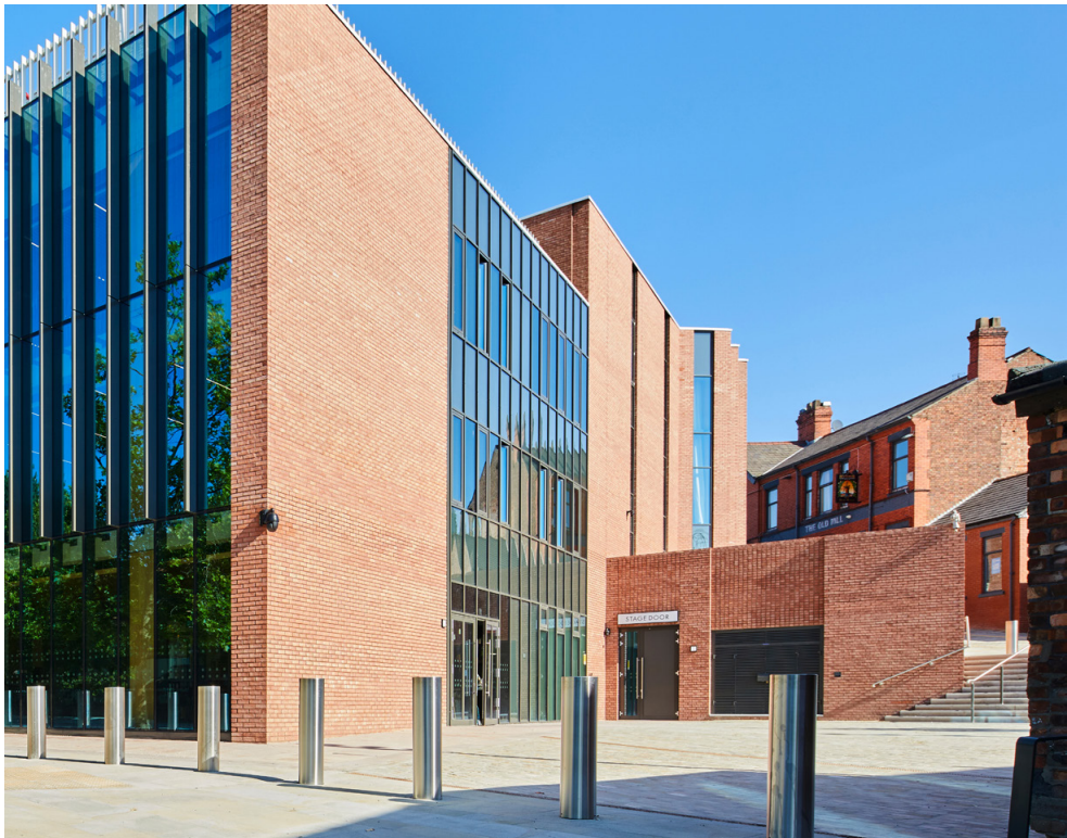
The substation seen from Prospero Place
