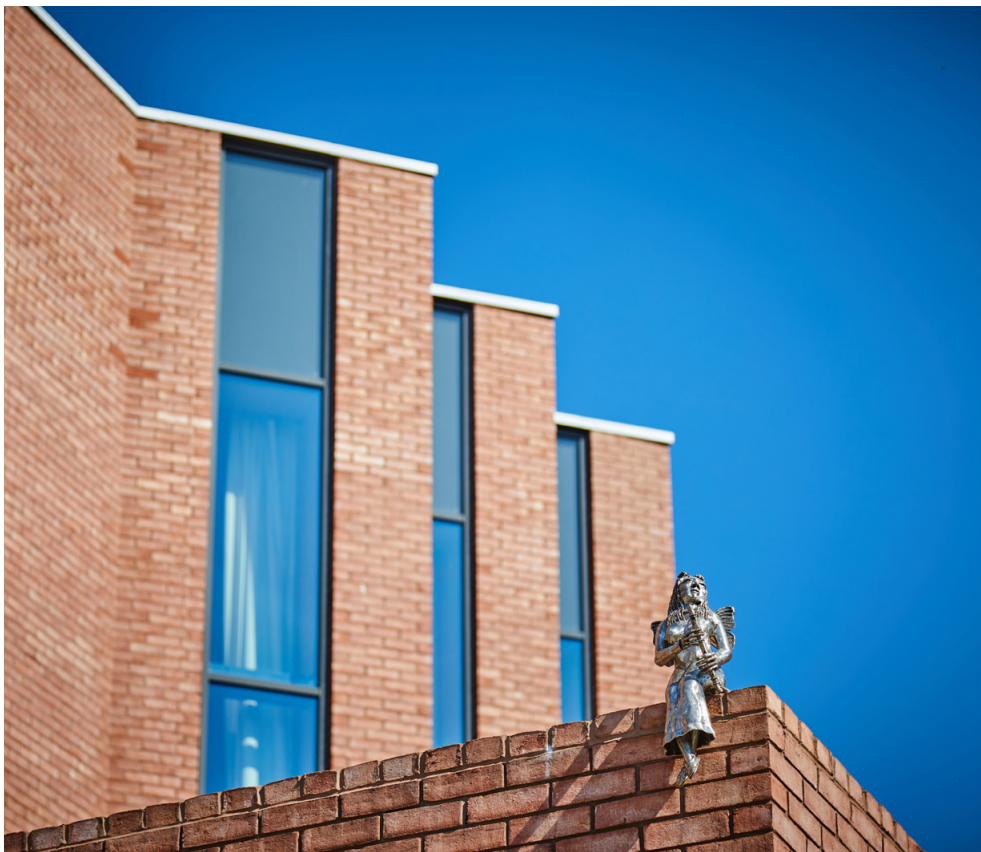
The edge of the substation roof with small sculpture
