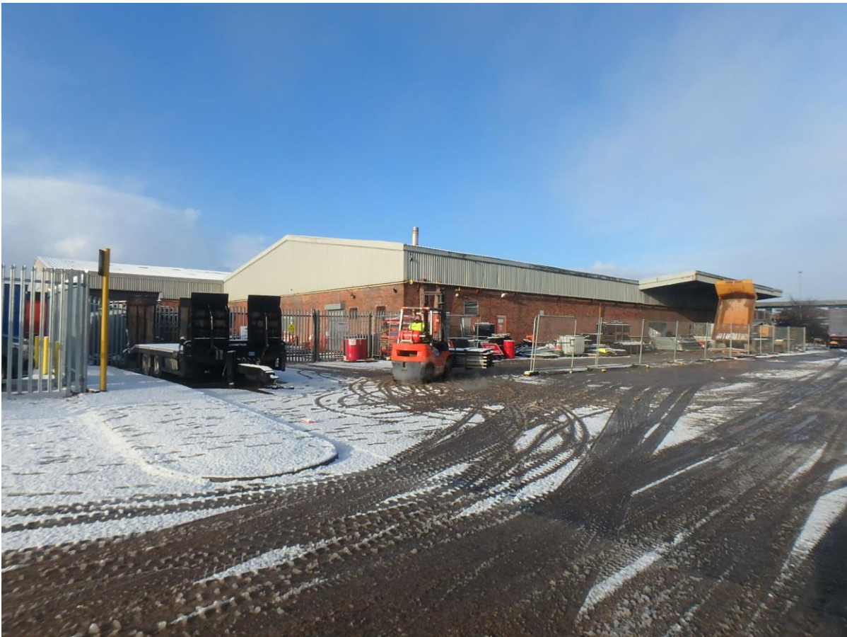
Unit 6 – South/East Elevation
