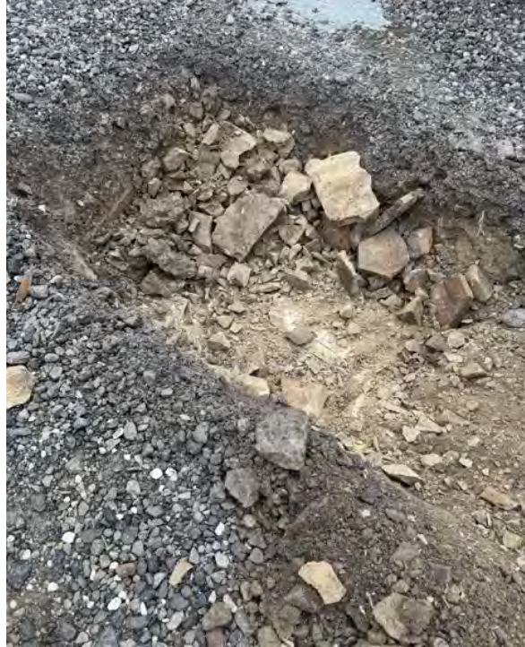
Photo 5: Trial pit showing mud stone to high level.
