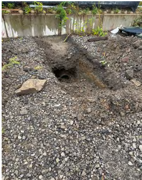
Photo 4: Exposed surface water pipe stub into site.
