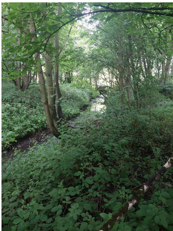
Photograph 7 – Ochre Brook within the woodland, showing culvert present at western extent of site.
