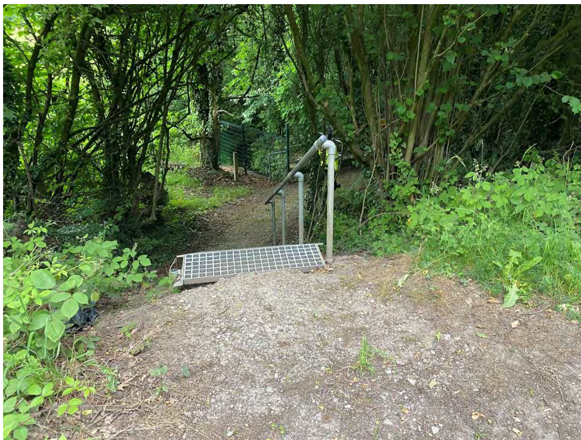
Figure 2.5: Steps leading down to water works.
