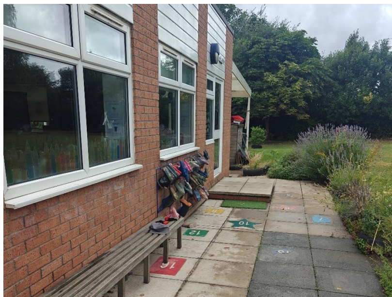
Existing stepped access to nursery classroom
