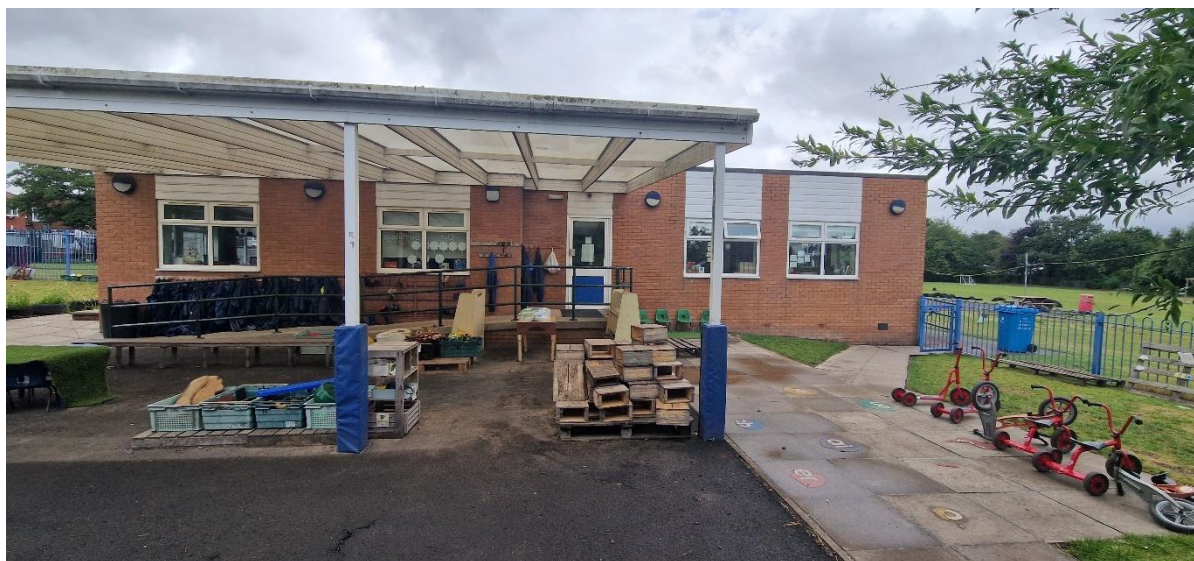
Existing covered play and access ramp to the external reception and nursery play area
