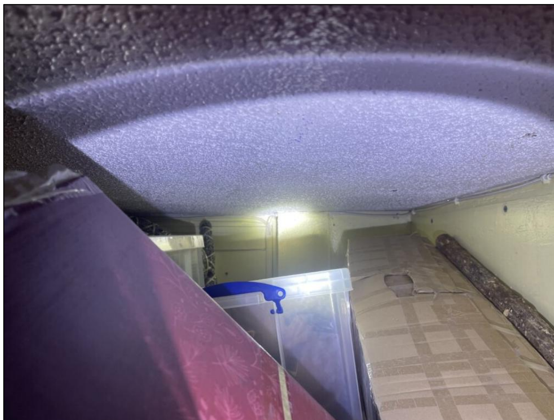
Plate 7 – Interior of the closet space identified in the hall, note this space has no access to the roof of the building
