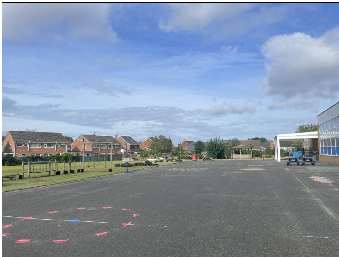
Plate 9 – Additional perspective of the exterior of the school, with note to amenity grassland and hardstanding present
