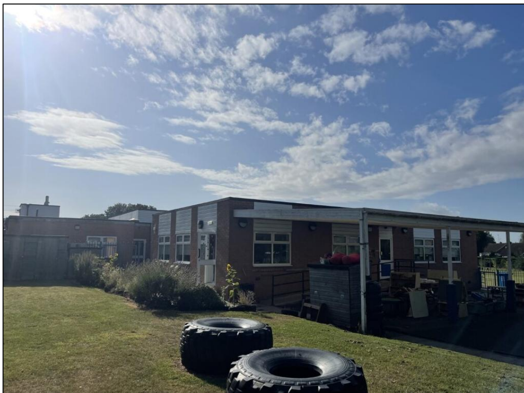
Plate 1 – South elevation of the school, showing the area of proposed works to the outdoor nursery area
