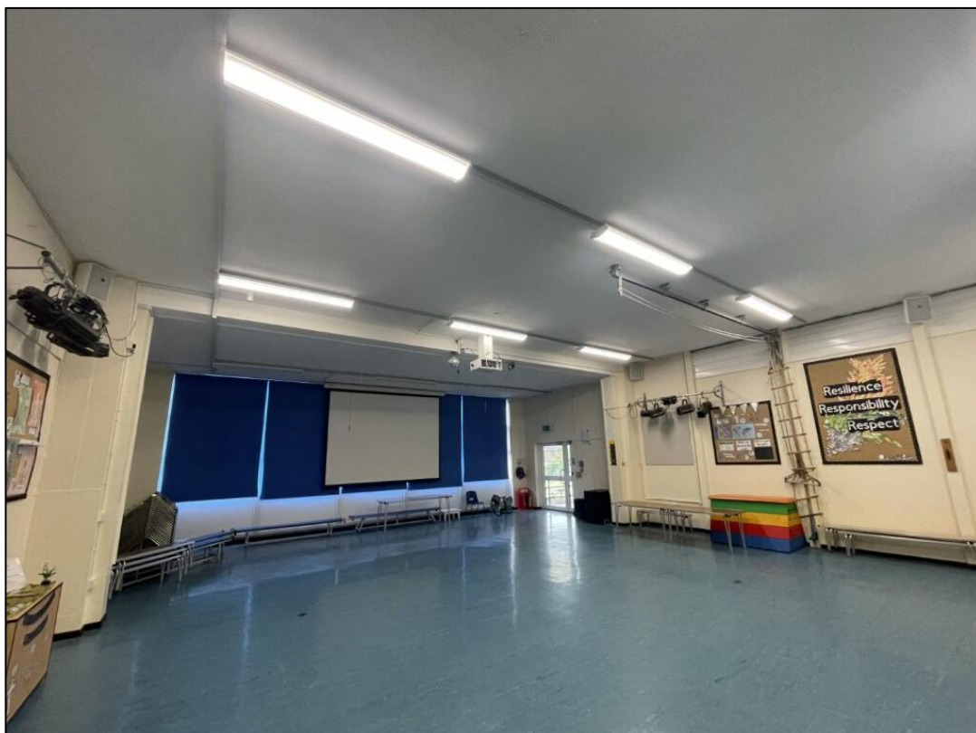
Plate 5 – Interior condition of the school hall, note this structure reaches to the roof with no loft space present
