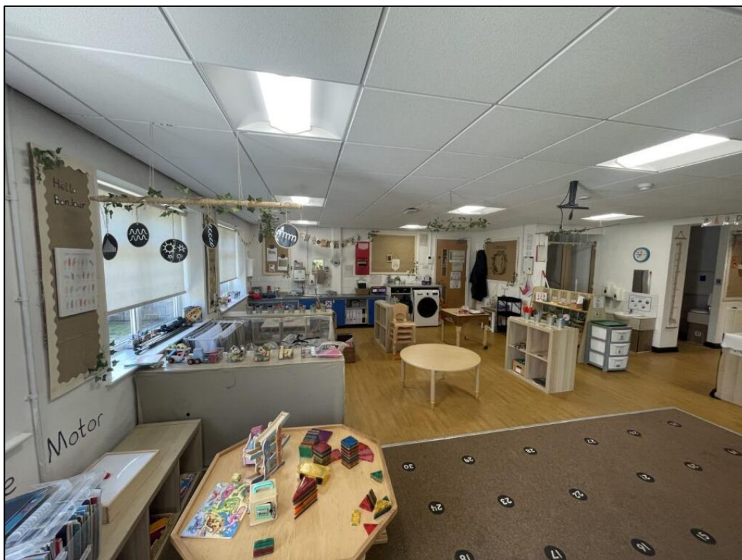
Plate 3 – General interior of the school building, note suspended flat ceiling with panels and fluorescent lighting used
