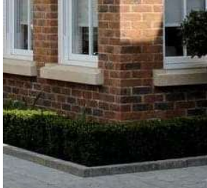
Stone window sills and heads
