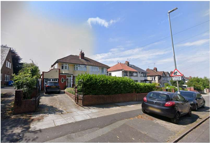
Properties along Church Road
