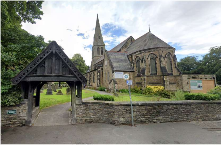
St. Bartholomew's Church
