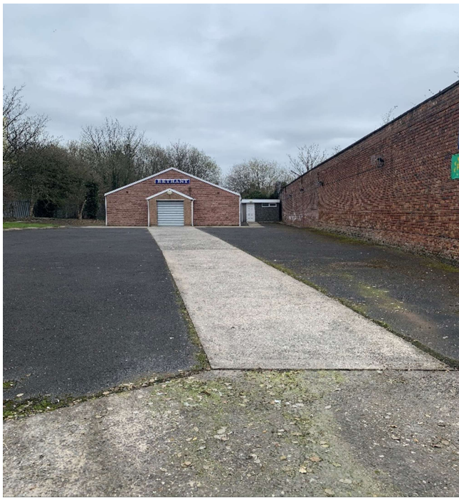
Fig. 7 View of Bethany Gospel Chapel and North Boundary wall
