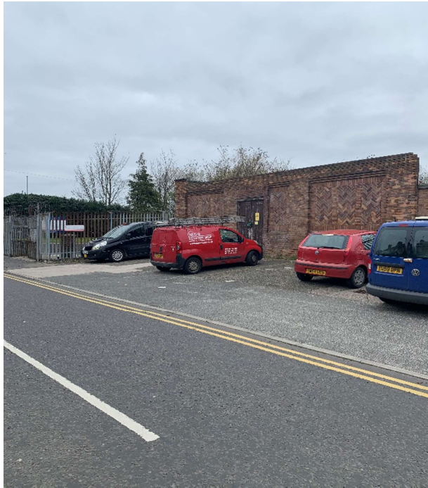
Fig. 4 View of sub station no longer in use – to be demolished
