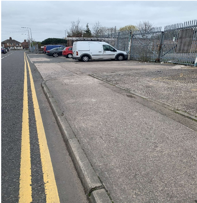
Fig. 4 View of site off Dinas Lane
