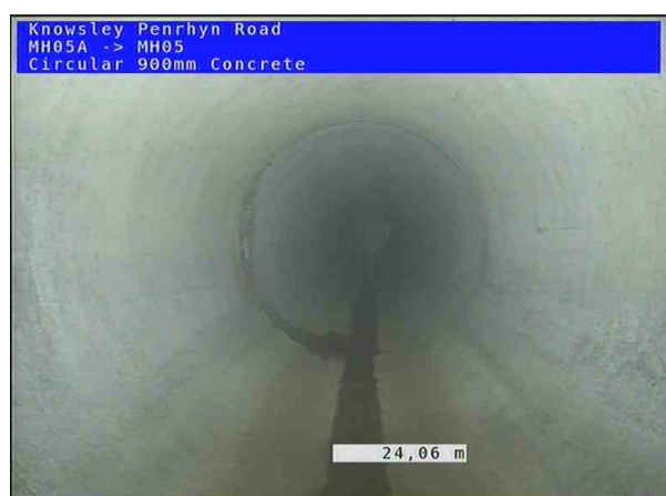
MH05A_9c5d008f-27e8-414a-9280-e5ffabfe89b0_20220427_144309_525.jpg, 00:02:09, 24.06 m General photograph taken at this point
