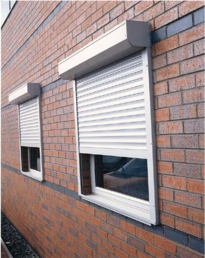
Photograph indicating: Proposed New external security roller shutters
