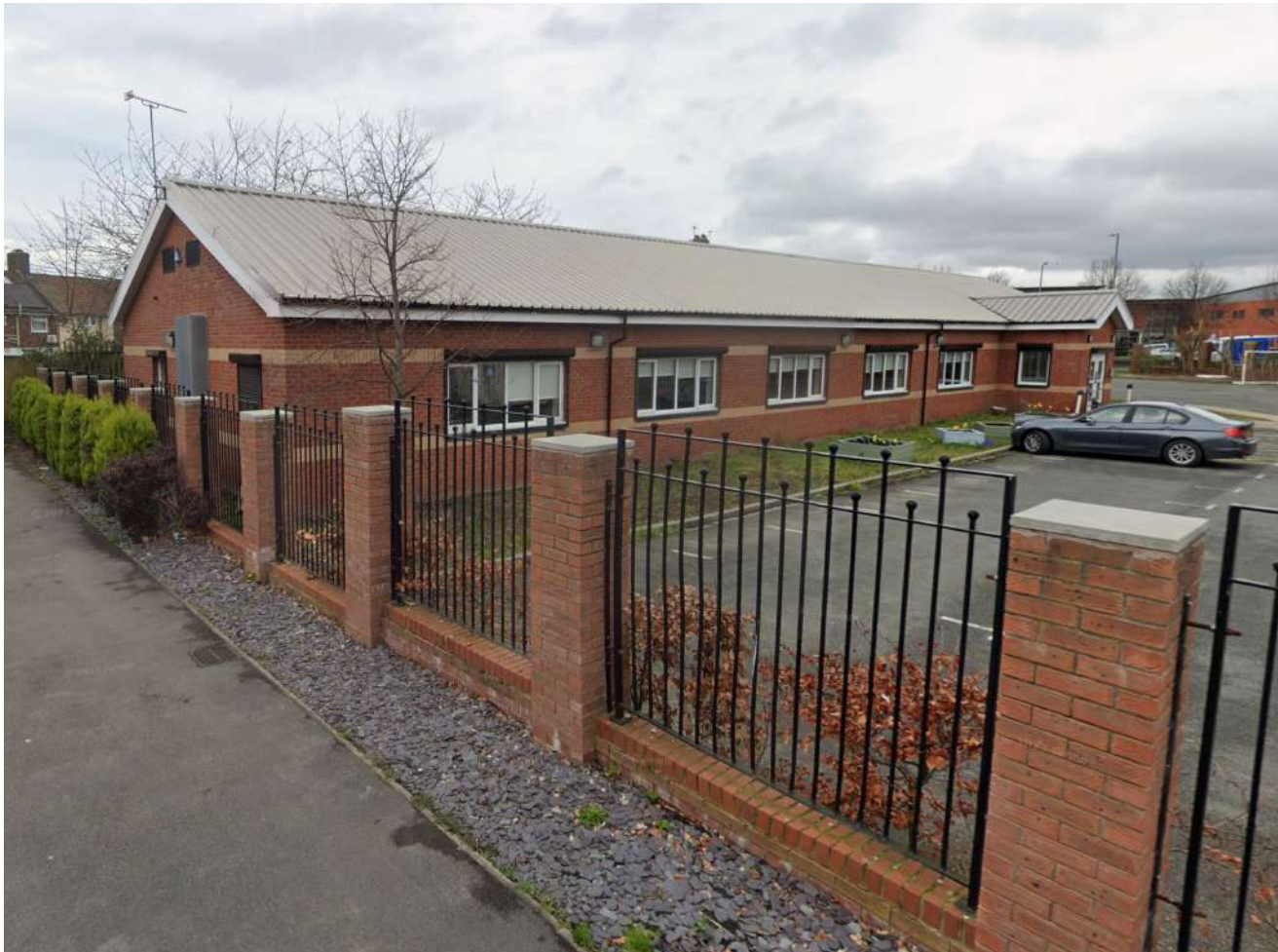
Photograph indicating: Existing external security roller shutters to be replaced -
