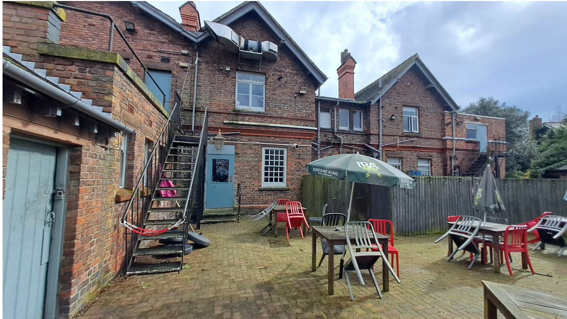
The rear of the building
