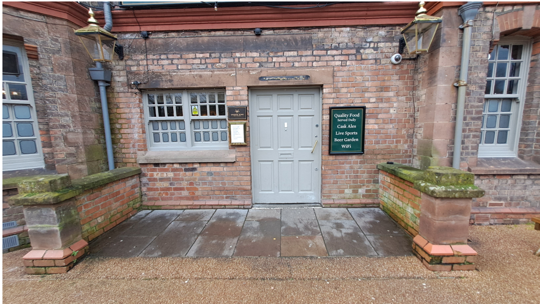
Front main entrance
