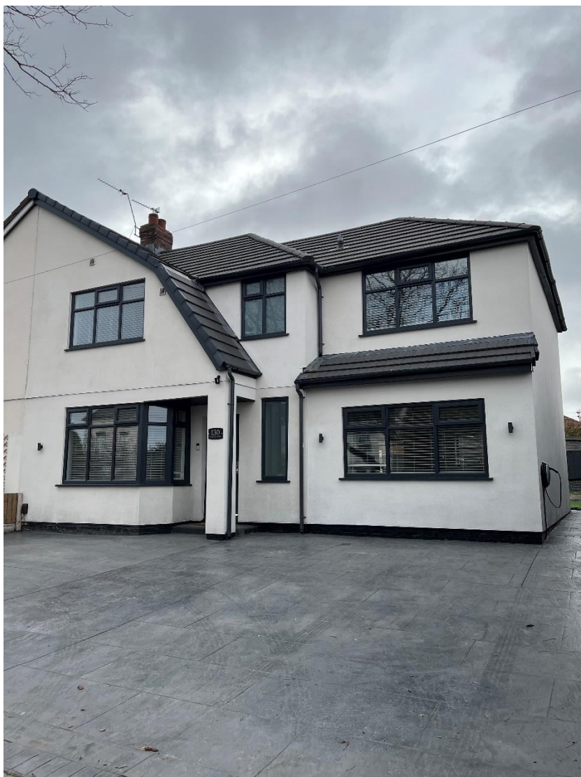
Front elevation of no.130.
