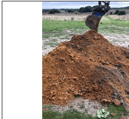
Trial Pit 101 Spoil
