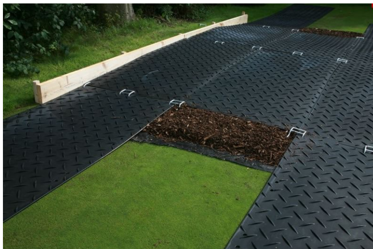
Figure 3. Ground protection interlinked plastic boards with a layer of wood chippings at least 150mm deep.
