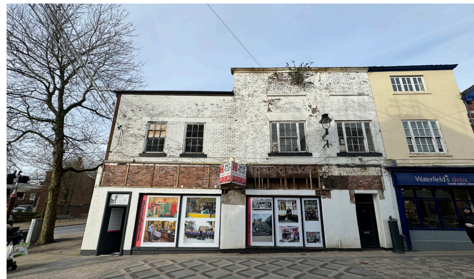
07. View of existing building on site
