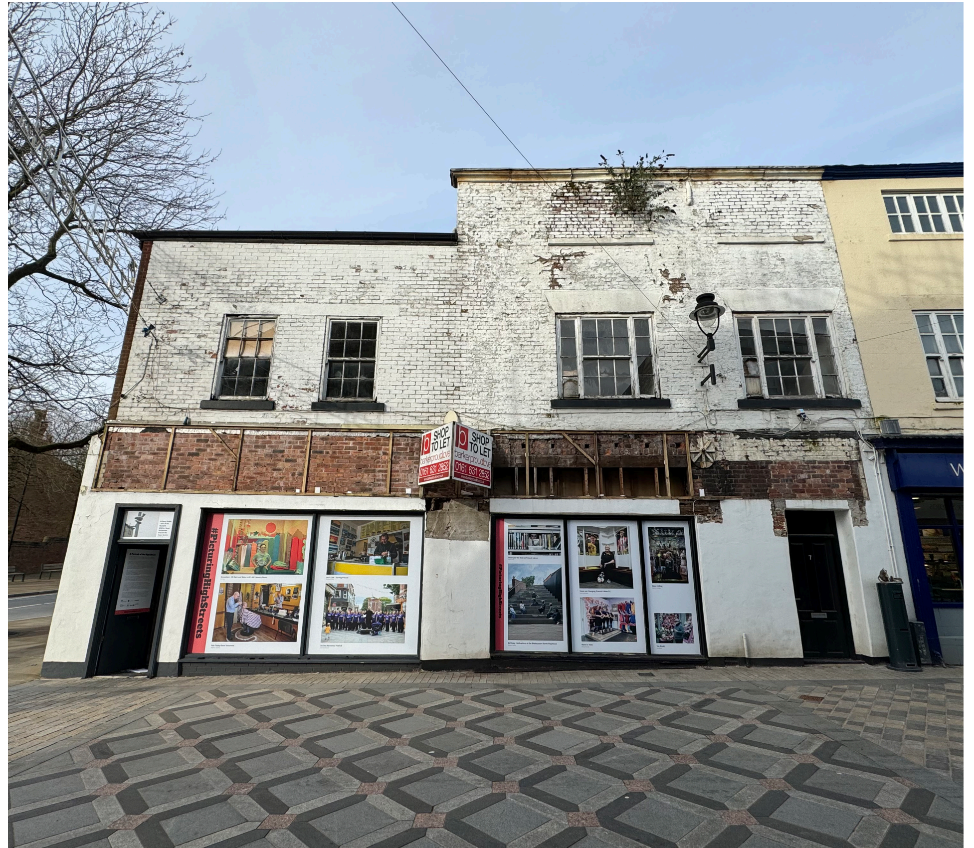
01. Photograph of existing building on site
