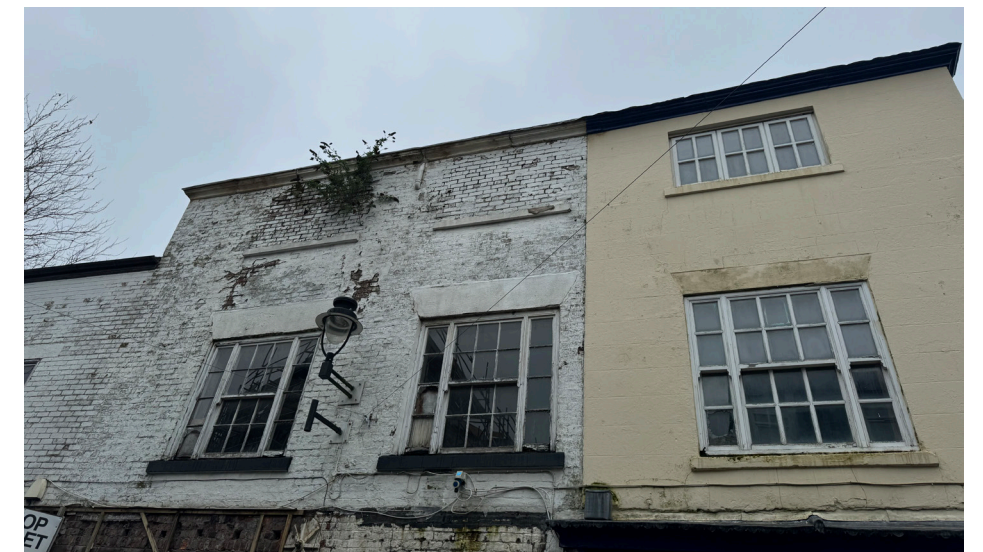
08. View of existing buildings condition
