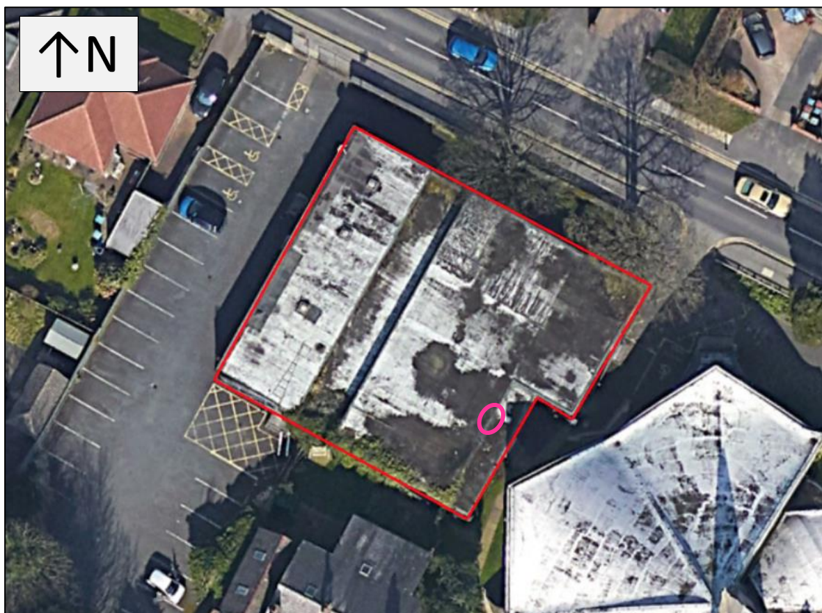
Figure 4.3 – Location of emergence point © Google Earth Pro 2025
