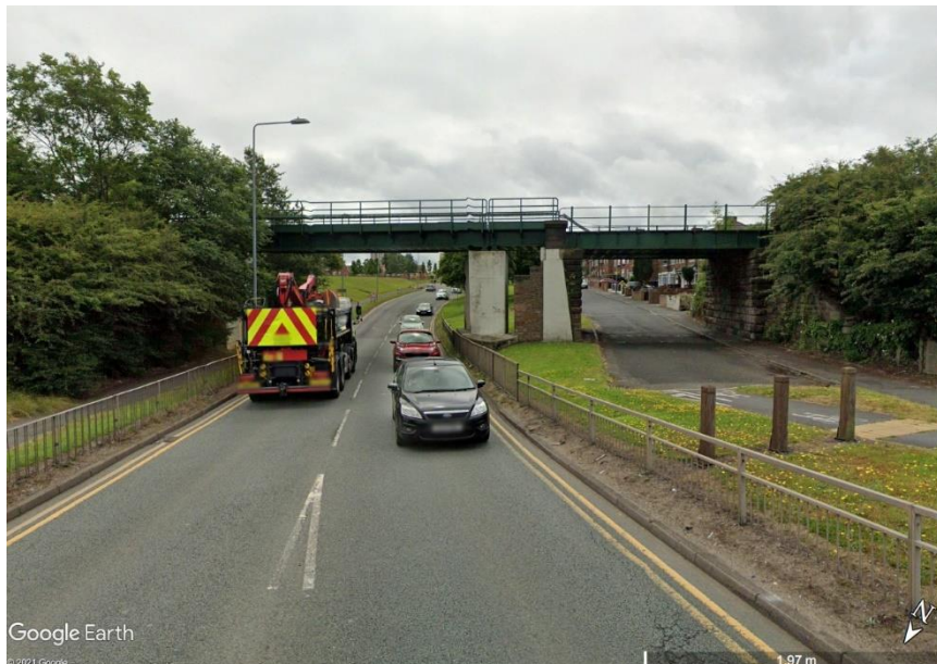
Photograph 6: Underbridge 55, looking south (Source: Google Earth)
