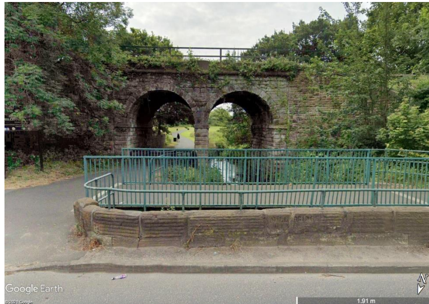
Photograph 5: Underbridge 56, looking south (Source: Google Earth)
