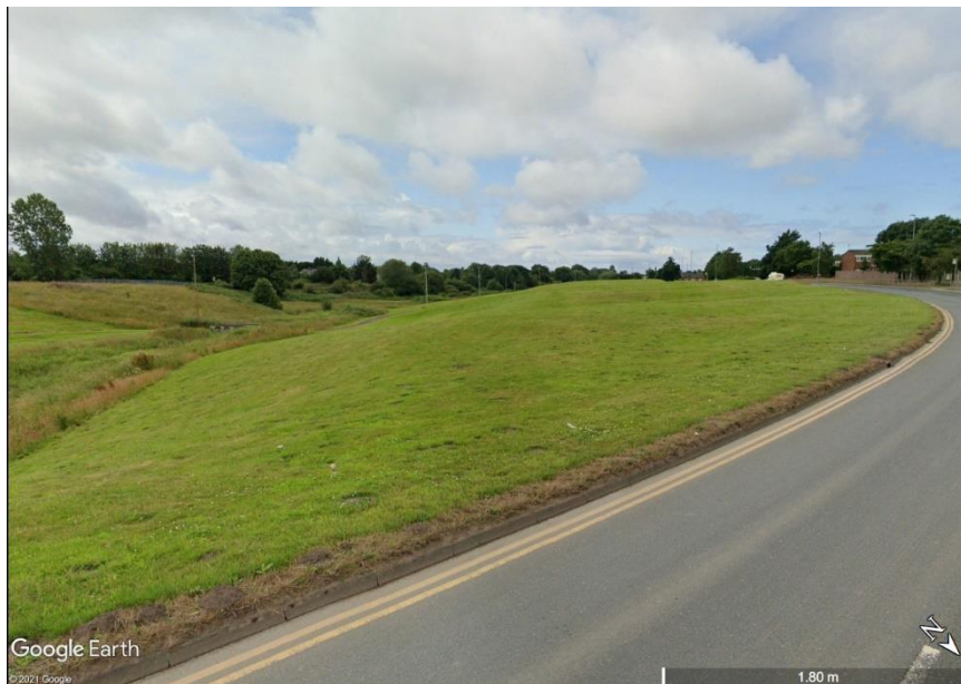
Photograph 4: View over the site of Tanpit House, looking south-west (Source: Google Earth)
