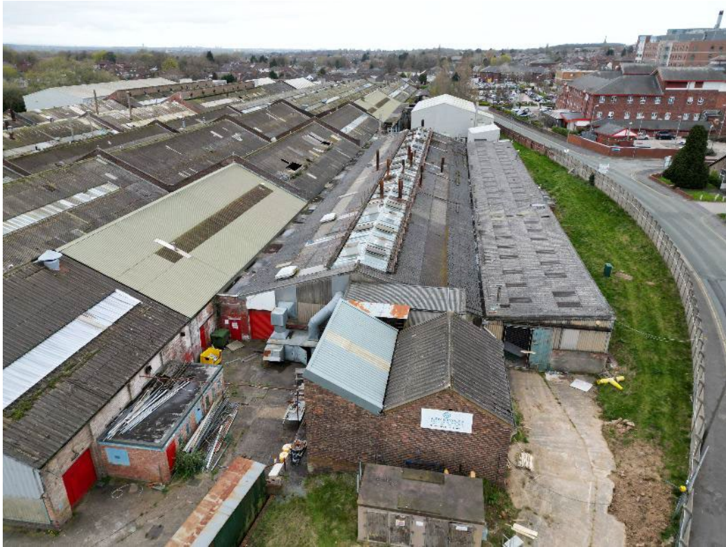
Plate 5. General view west/north-west across the study site © Urban Regen
