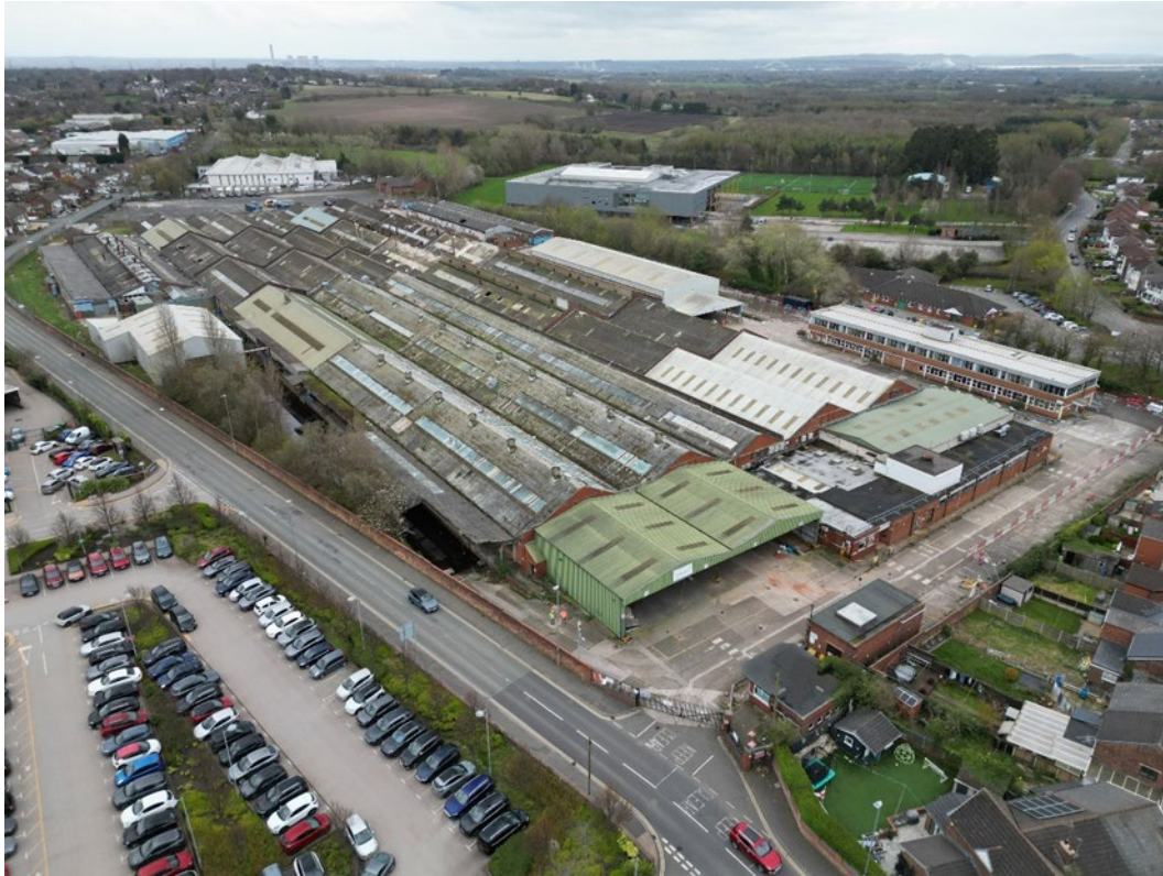
Plate 1. General aerial view south—east across the study site © Urban Regen
