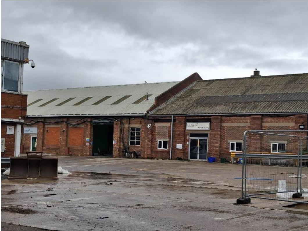
Plate 13. View north/north-east of part of the southern elevation of Building B1
