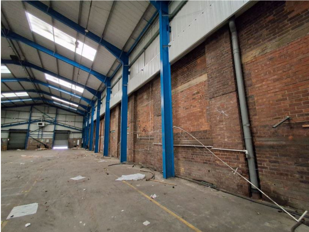
Plate 15. View within Building B1 of an exterior wall, highlighting a modern steel structure which has been erected within, supporting the pitched roof.
