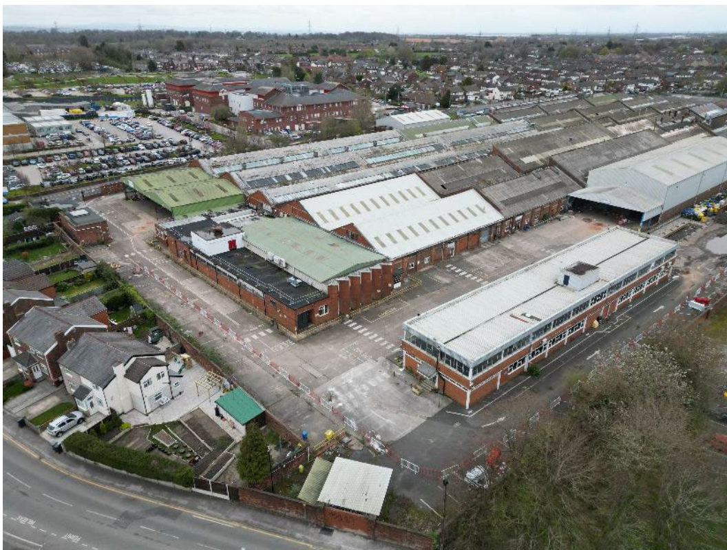
Plate 2. General aerial view north-east across the study site © Urban Regen
