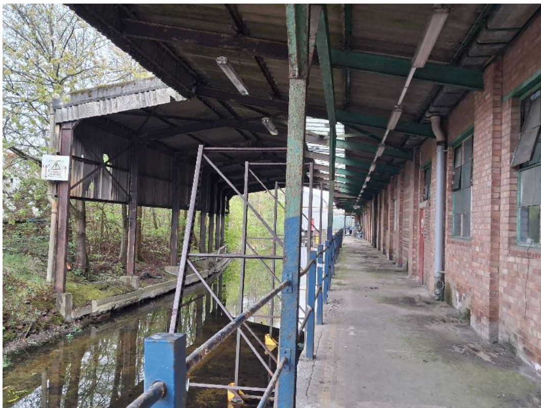
Plate 14. View west/south-west along the northern elevation of Building B1, along the elevated platform.
