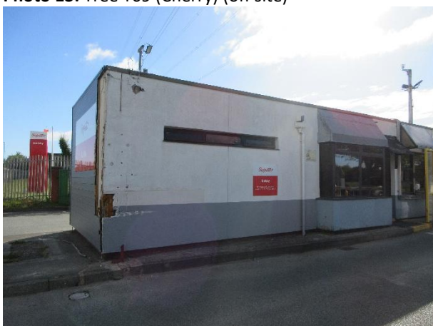
Photo 15: Northern and western elevations of the gatehouse
