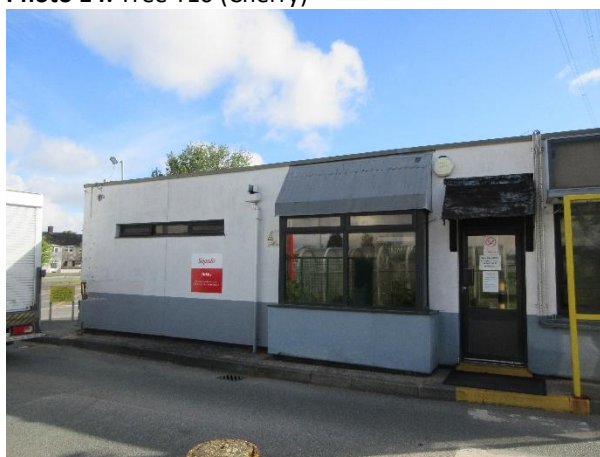
Photo 16: Western elevation of the gatehouse
