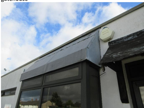
Photo 17: Sealed material over canopy at gatehouse
