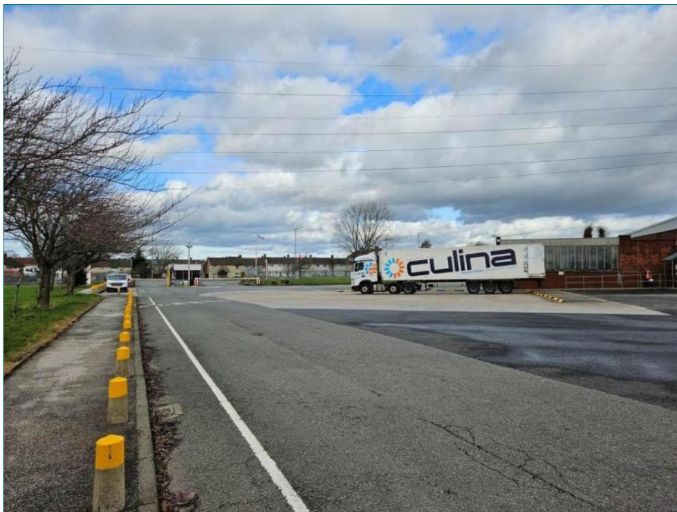
Photograph 5: Looking Northwest Towards the Entrance to the Site.
