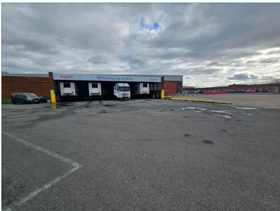
Photograph 4: Looking East Towards the Existing Building.
