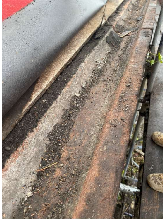
Plate 7 – Drainage channel to stone gutter blocks to the northwest roof slope.
