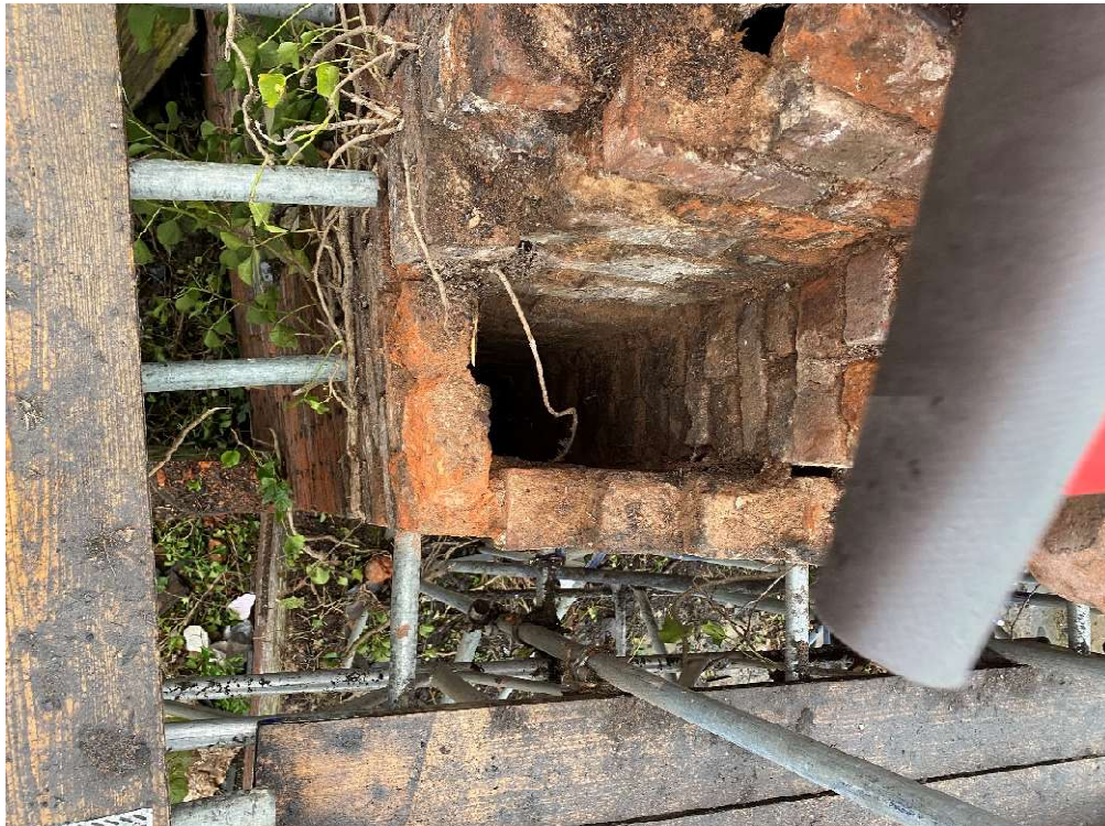
Plate 6 – Internal stack to the northeast corner of the northwest elevation.
