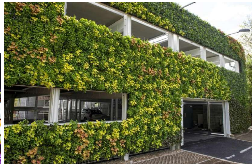
Pre-constructed National Grid Car Park, Leamington Spa (built in four weeks)
