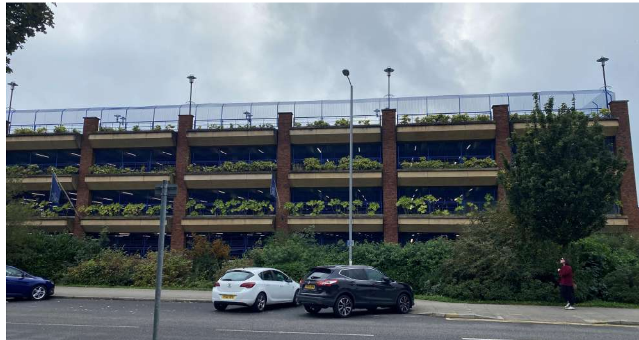
Retrofitted Millgate Shopping Centre Car Park, Bury
