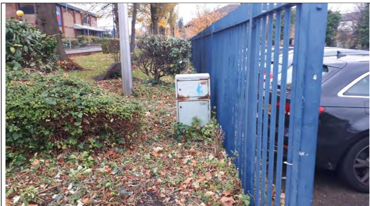
Photo 29 – Boundary of car park
