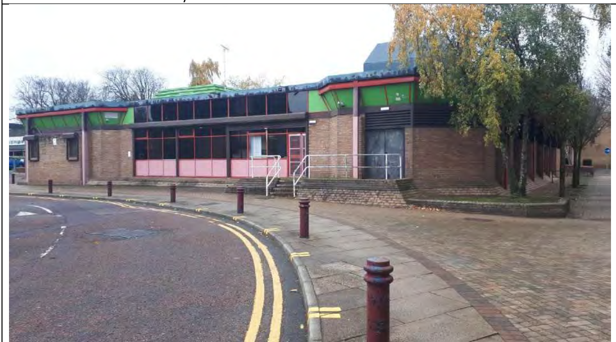
Photo 10 – Council building located in the south east corner of the site
