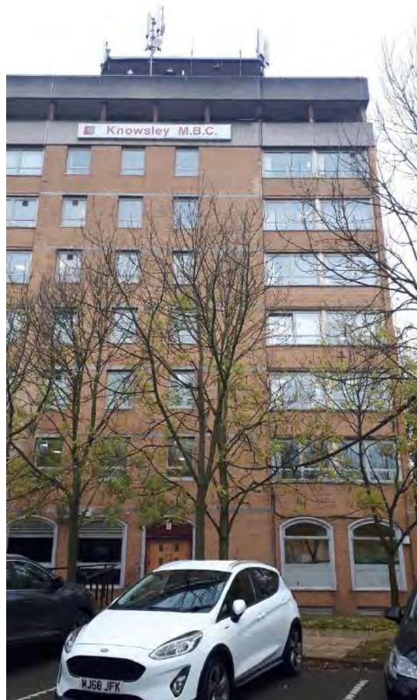
Photo 6 – Knowsley Council building located on site
