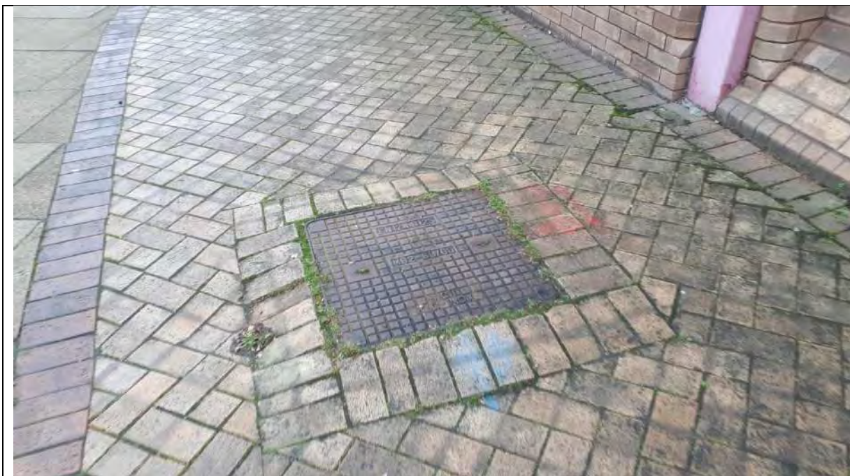
Photo 11 – Evidence of services on site
