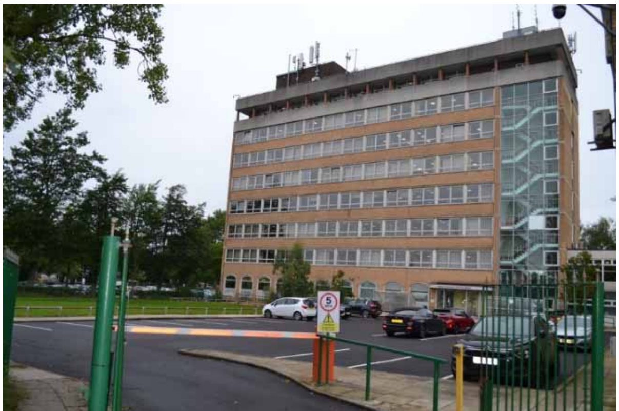
Plate 39: Sightline to the north-east highlighting the south-west facing elevation of the Council Municipal Building.
