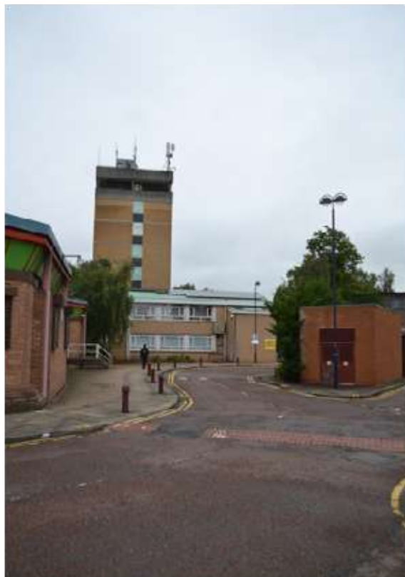
Plate 20: Sightline to the along Westmorland Road with the north-facing elevation of the Council Municipal Building prominent.
