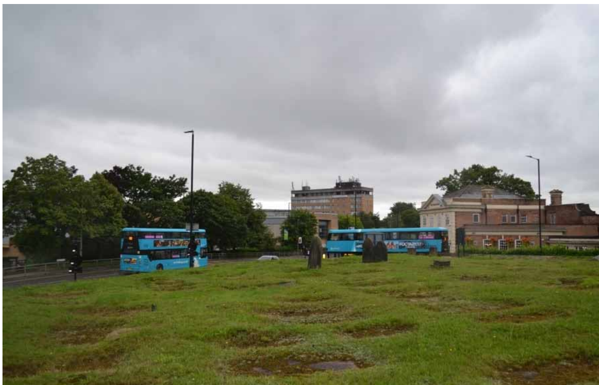
Plate 2: Sightline to the south towards the Site from the churchyard of St. Michael's Church, Listed Building (Grade II*, NHLE ref. 1075535). The eight-storey Council Municipal Building is prominent and acts as a sky-lined eye-catcher.
