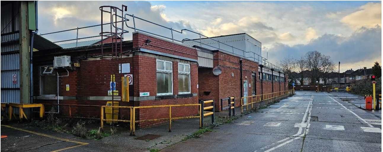
Image 1C(1) – Building 1C exterior viewed from the north west
