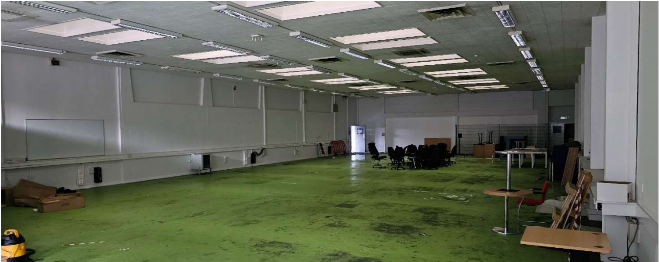
Image 1C(4) – Building 1C portal frame interior
