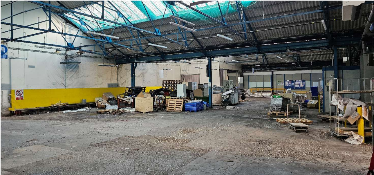
Image1D(2) – Interior of the western end of Building 1D (main building) with the fabric wall evident
