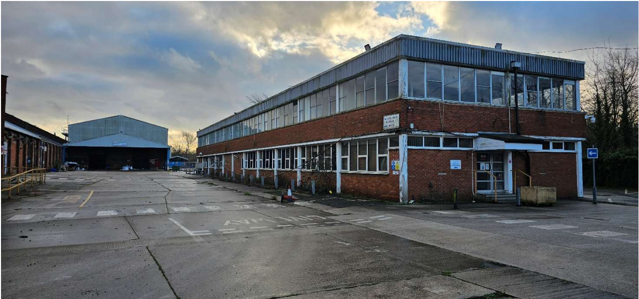
Image 1G(1) – Building 1G exterior viewed from the west
