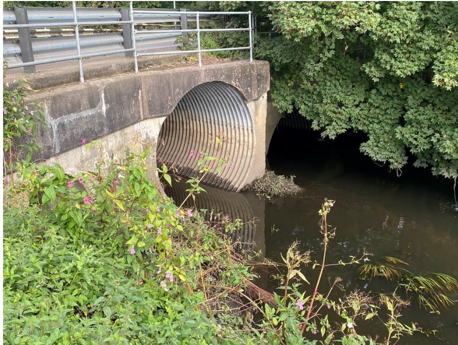
Photograph 7: Greensbridge Lane Structure IMG_2764.JPEG. Photo looking upstream
