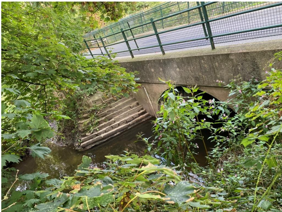
Photograph 2: Cartbridge Lane Structure IMG_2772.JPEG. Photo looking upstream
