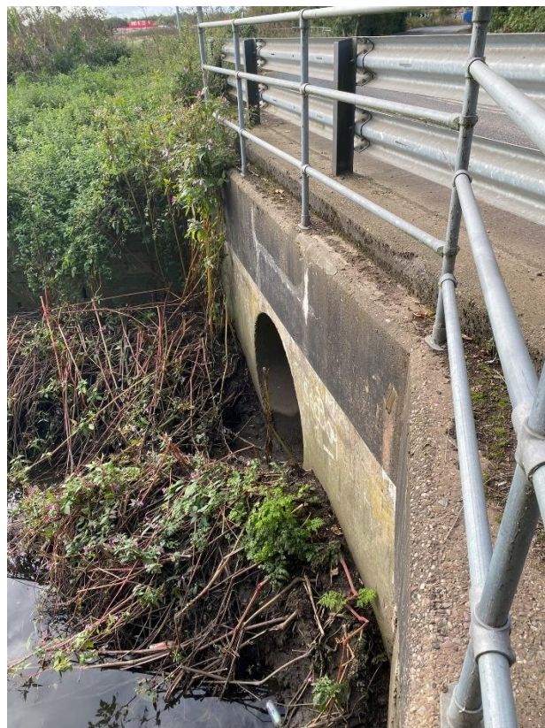
Photograph 8: Greensbridge Lane Structure IMG_2769.JPEG. Photo looking upstream
