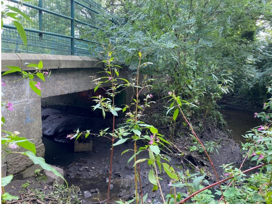
Photograph 3: Cartbridge Lane Structure IMG_2776.JPEG. Photo looking upstream
